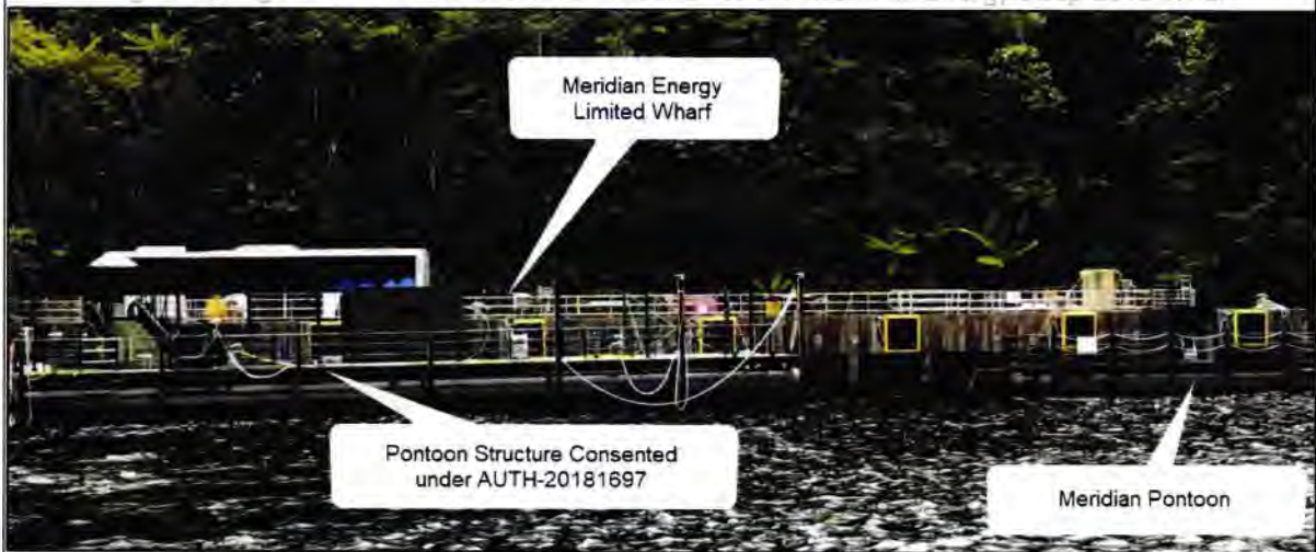
Image showing the location of structures attached to the Meridian Energy Deep Cove Wharf
