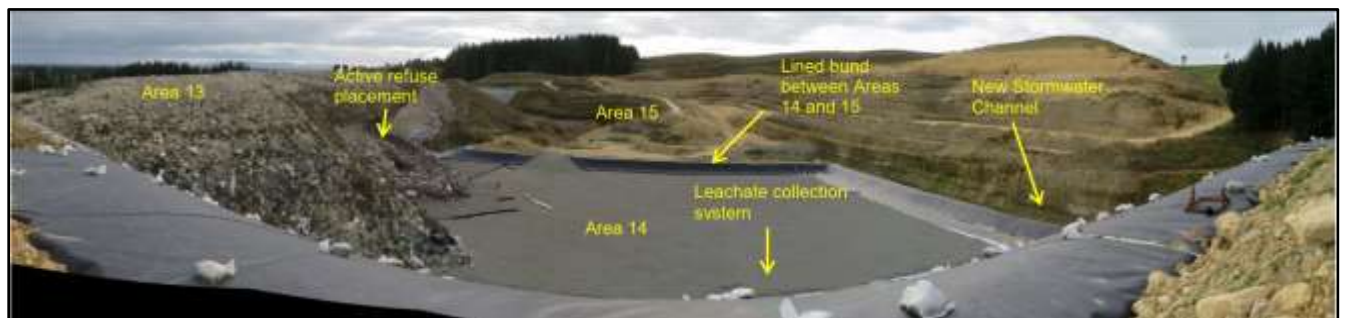
Figure 5: Historic photo of the view looking west across Areas 13, 14 and 15 showing the liner and bund between Area 14 and 15
