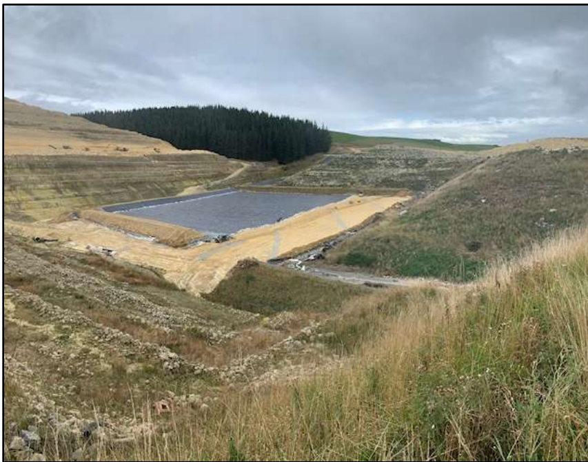
Figure 2: Area 15 construction progress as at week of the 06/04/2020
