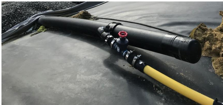
Figure 21 Leachate clean-out pipes extended up the eastern side wall of the landfill (dated 01 August 2019).
