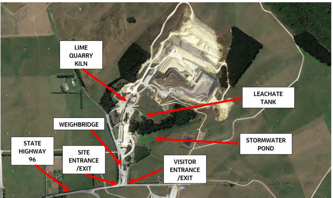
Figure 2 Close up of the AB Lime Landfill and Quarry
