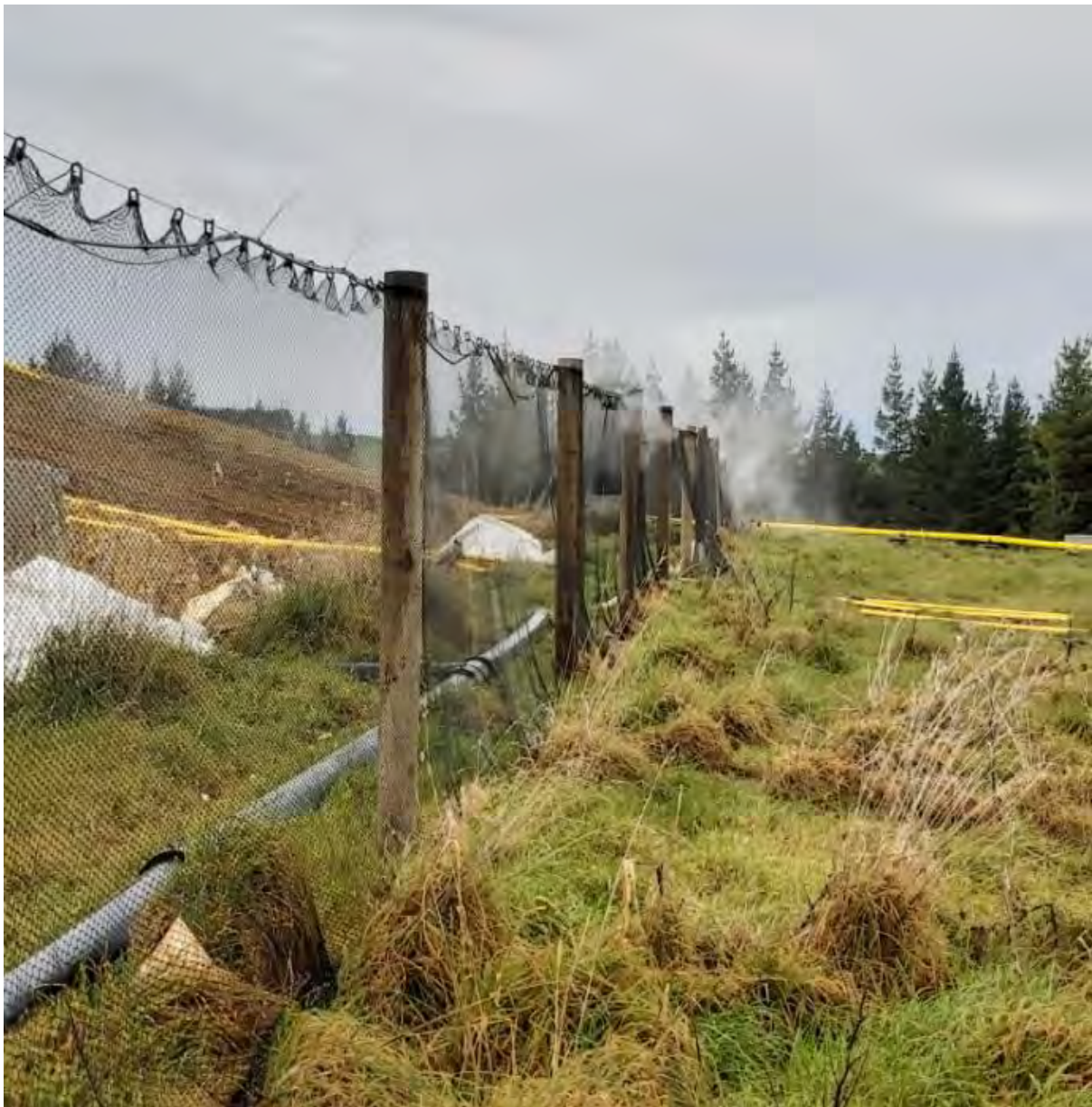
Figure 1. – Odour neutralising fence line spray system.
