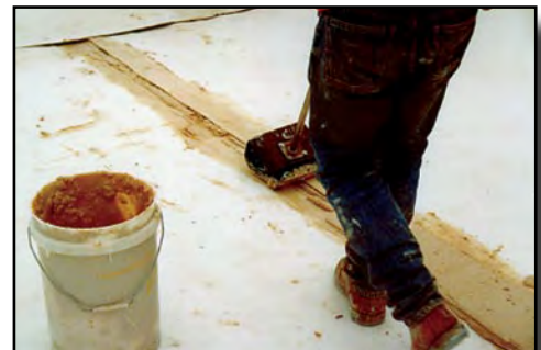
Applying the bentonite Fillet
