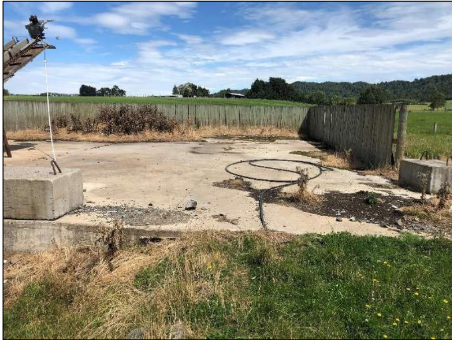
Figure 2.4: Weeping wall and solid storage area.
