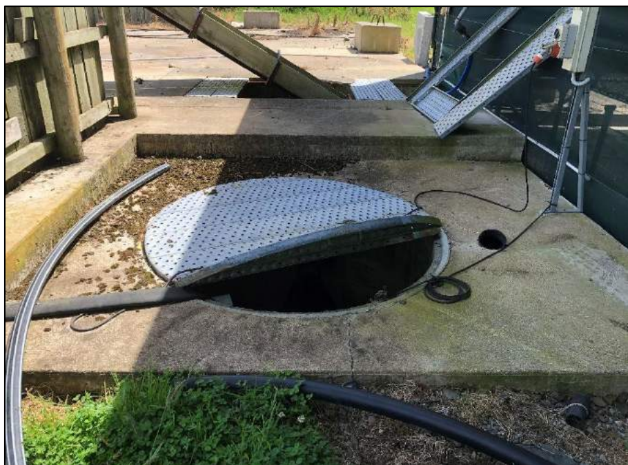
Figure 2.5: Transfer sump 1 at north-east corner of barn.
