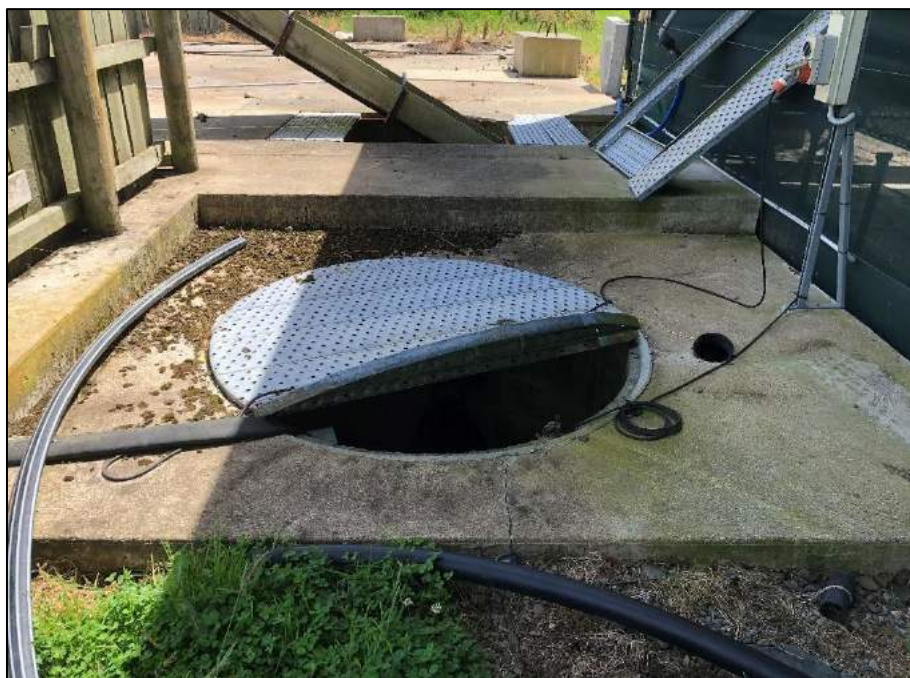
Figure 2.5: Transfer sump 1 at north-east corner of barn.
