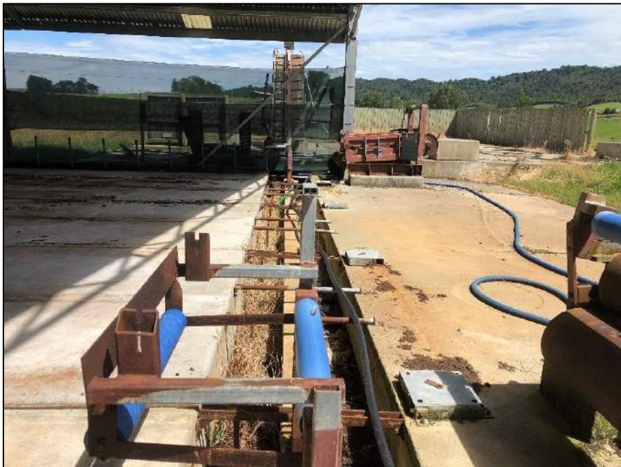
Figure 2.3: Conveyor chain and weeping wall.
