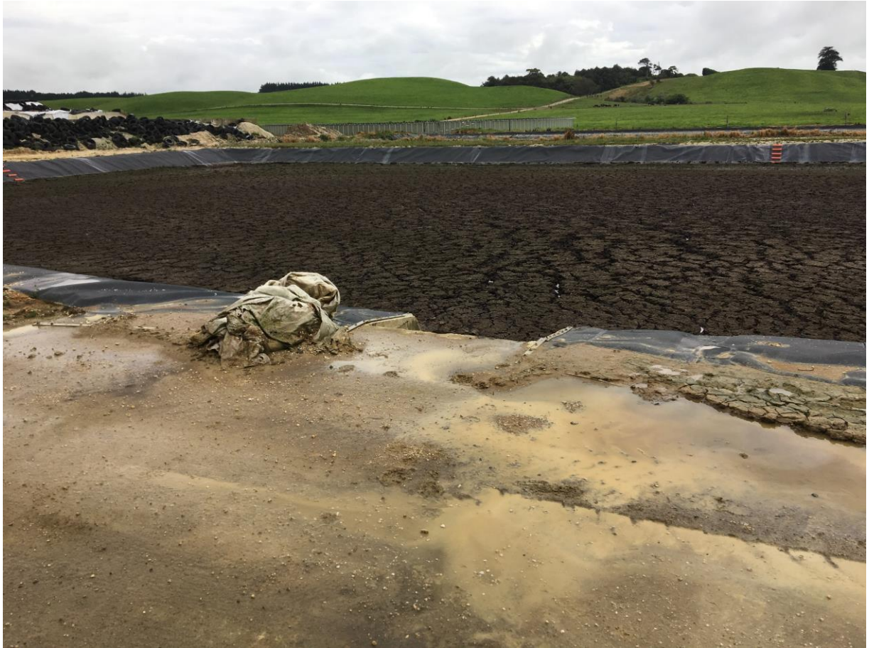
Picture 7: Wintering barn and solid scraping pond, with effluent pond 1 & 2 in the background. Wintering Barn and solids scrapings pond is emptied via slurry tanker.
