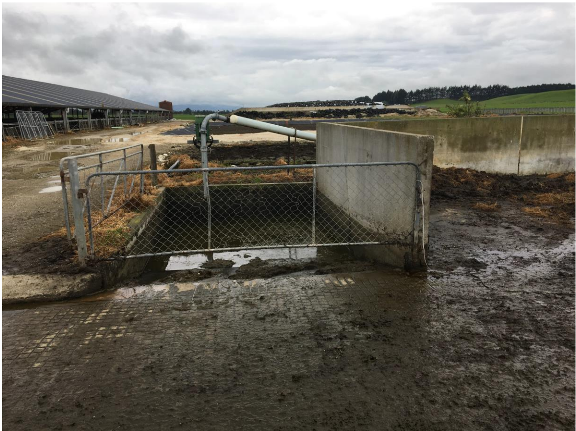
Picture 4: Sand trap located at the southern entry and exit point to the wintering barn.
