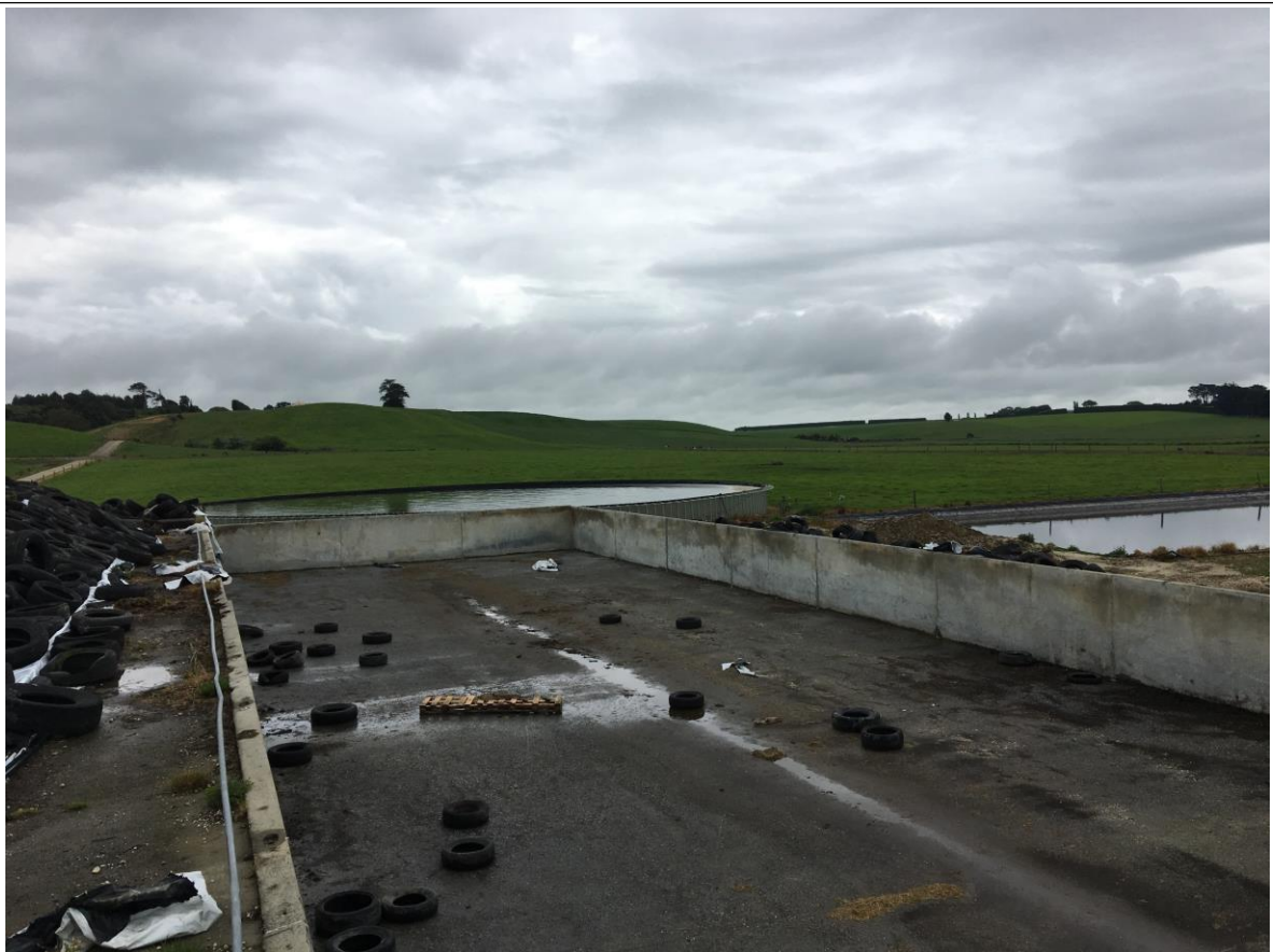
Picture 8: Dual silage pit with drains located throughout which flow to silage leachate sump located on the north eastern end of the shed. Silage leachate is discharge to land as a permitted activity under rule 41 of the pSWLP.
