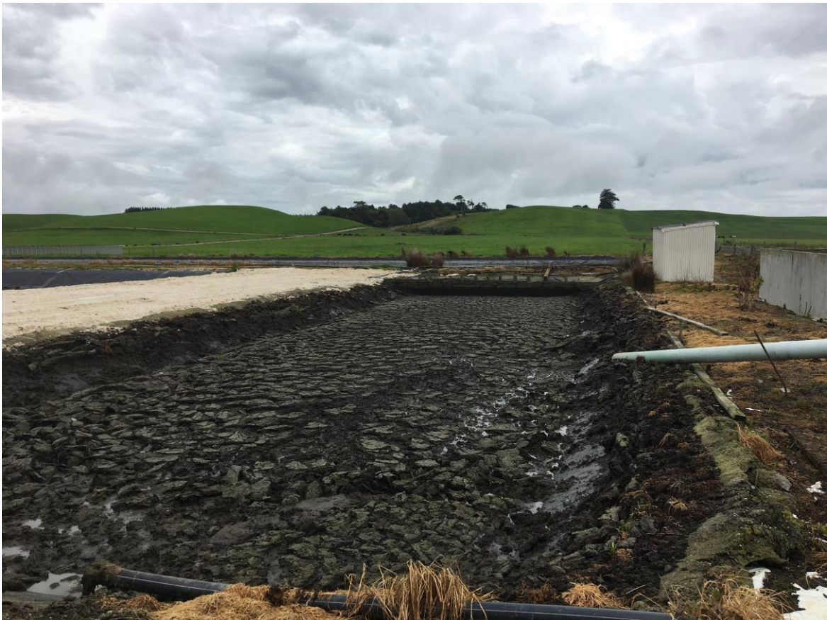
Picture 6: Weeping Wall, solids removed are spread to land as a permitted activity under Rule 38 of the pSWLP.
