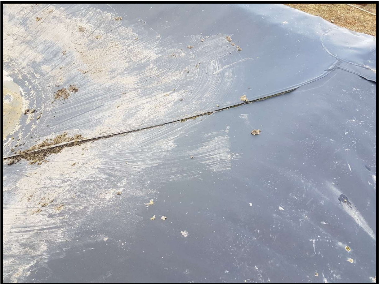
Figure 6 : Liner Seam Example
