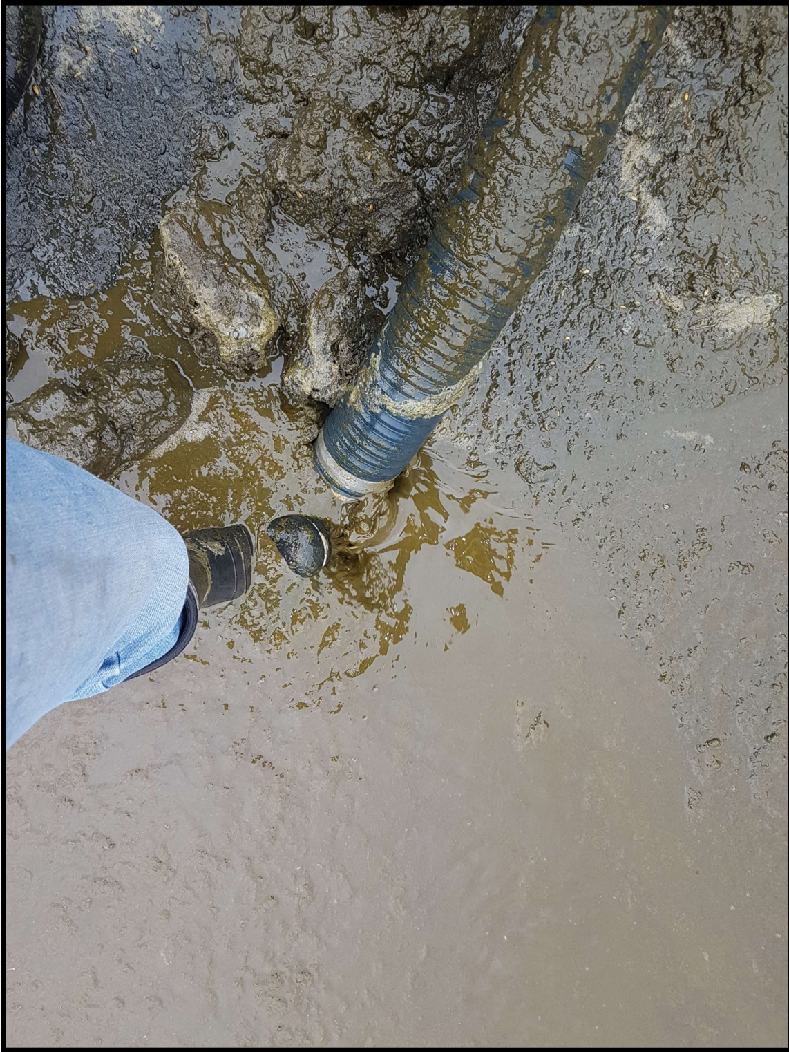
Figure 3 : Slurry tanker suction - showing depth of remaining effluent
