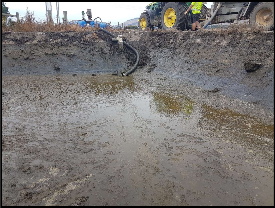
Figure 4 : South and west sump embankments
