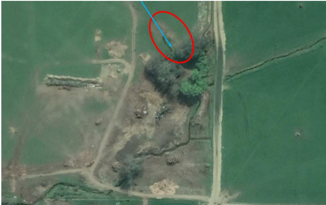
Figure 6: Aerial image from September 2018. CSA shown in red. Overland flow path shown in blue.
