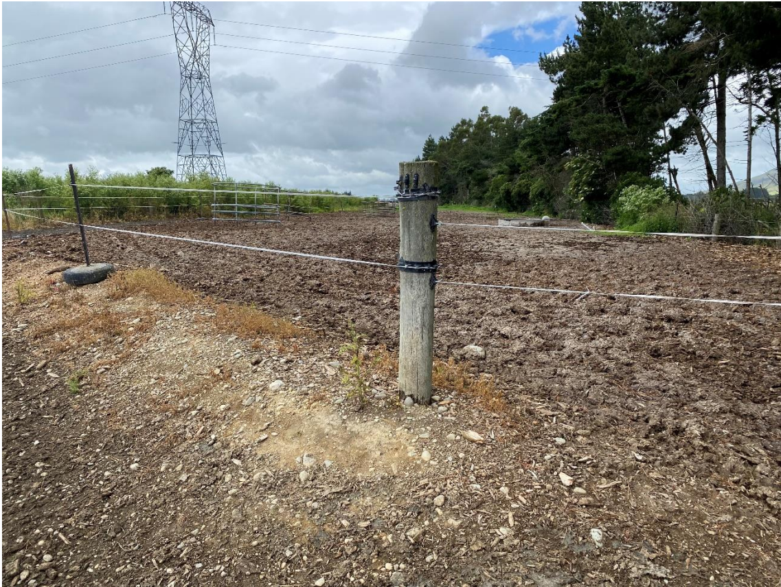
Figure 1: Gravel nibbing around calving pad. 500mm of woodchip/bark will be put on the calving pad prior to the pad being used.
