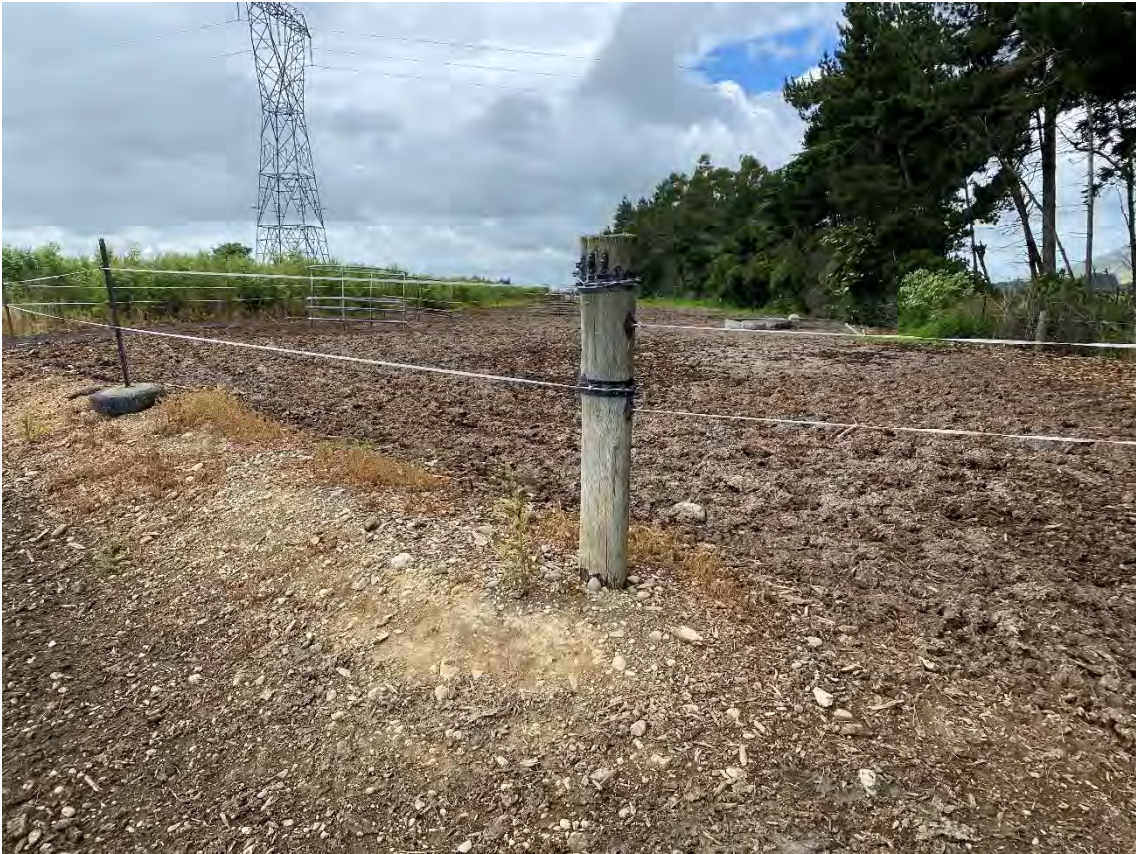
Figure 1: Gravel nibbing around calving pad. 500mm of woodchip/bark will be put on the calving pad prior to the pad being used.
