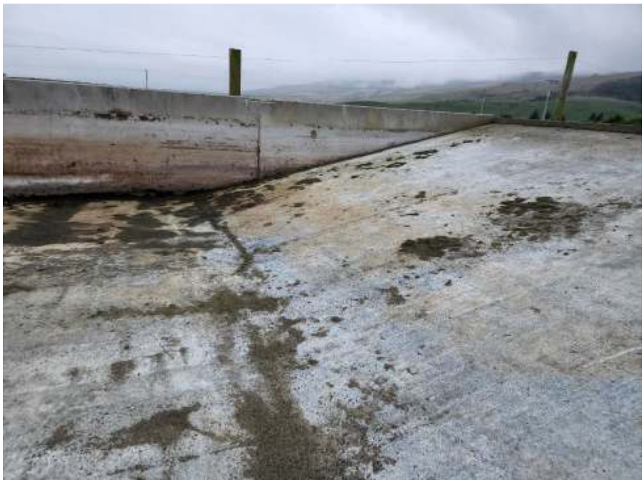
Figure 11 Interior of north sludge bed.
