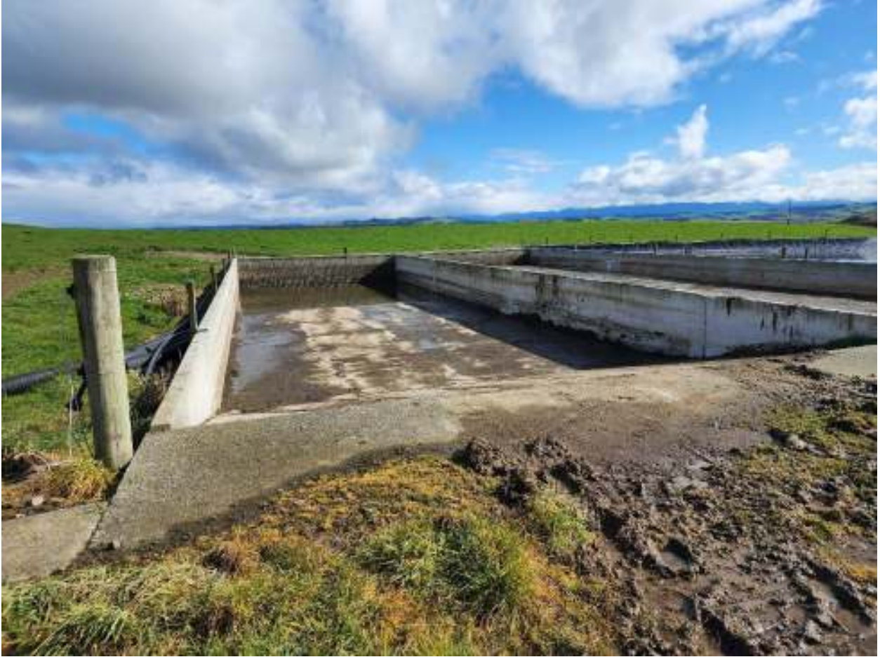
Figure 33 Interior of south sludge bed.
