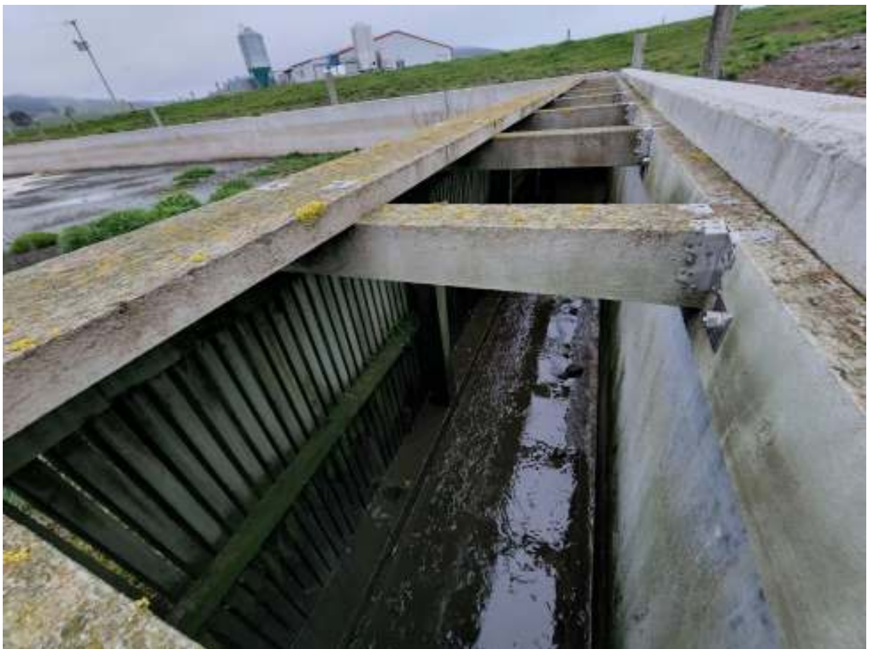
Figure 7 Interior of weeping wall structure.
