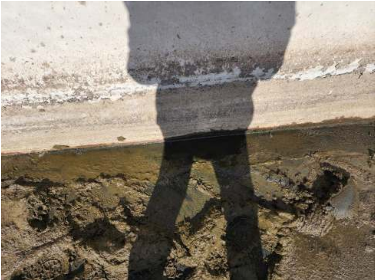
Figure 37 Edge join of south sludge bed.
