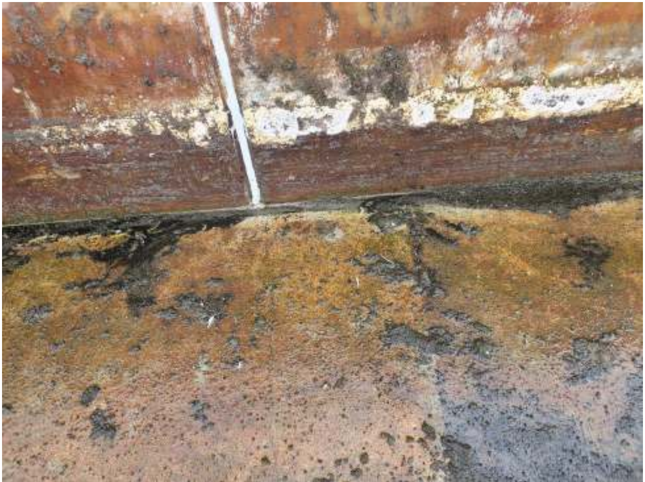
Figure 27 Panel joints of north sludge bed with repaired sealant.
