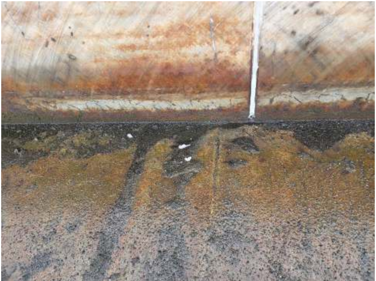
Figure 24 Panel joints of north sludge bed with repaired sealant.
