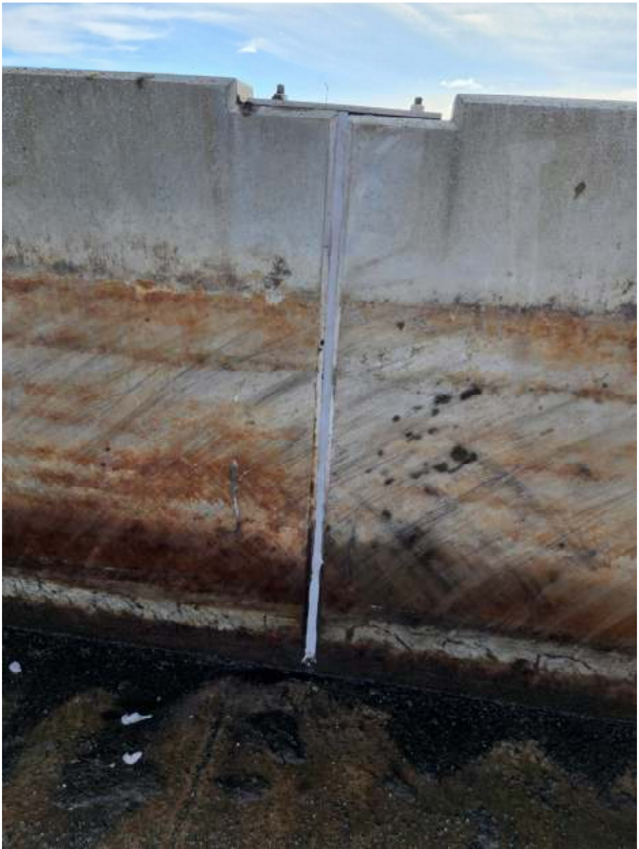
Figure 23 Panel joints of north sludge bed with repaired sealant.
