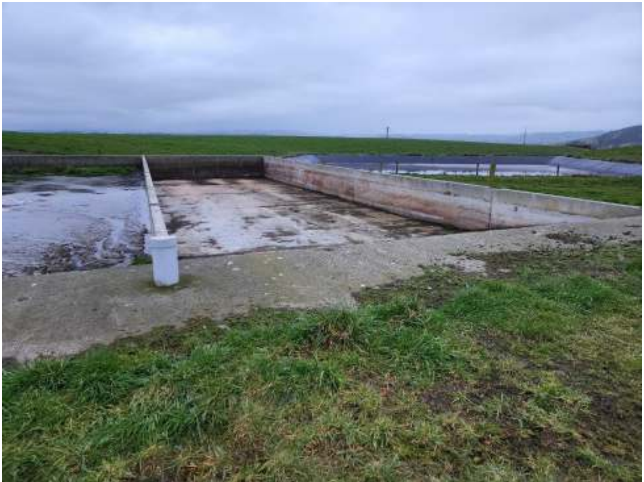
Figure 8 North sludge bed.
