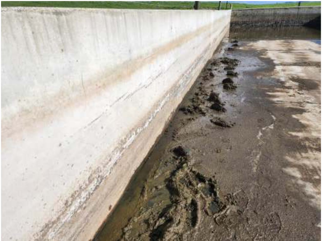
Figure 36 Edge join of south sludge bed.
