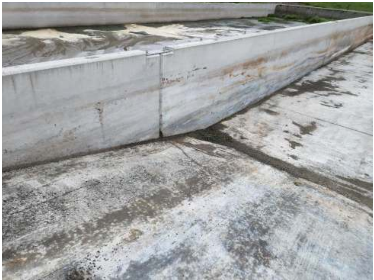
Figure 10 Interior of north sludge bed.
