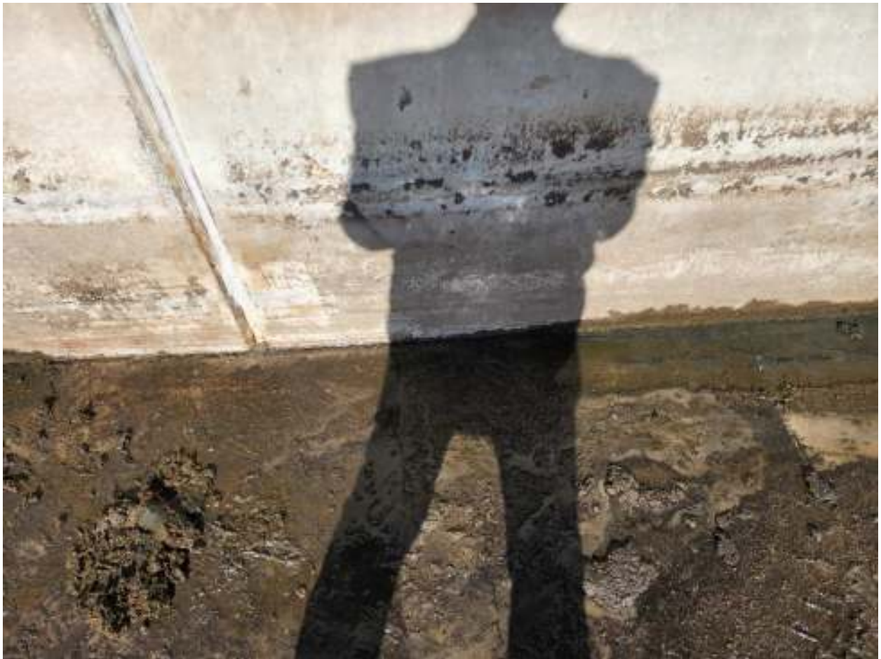
Figure 42 Panel joints of south sludge bed with repaired sealant and edge joint.
