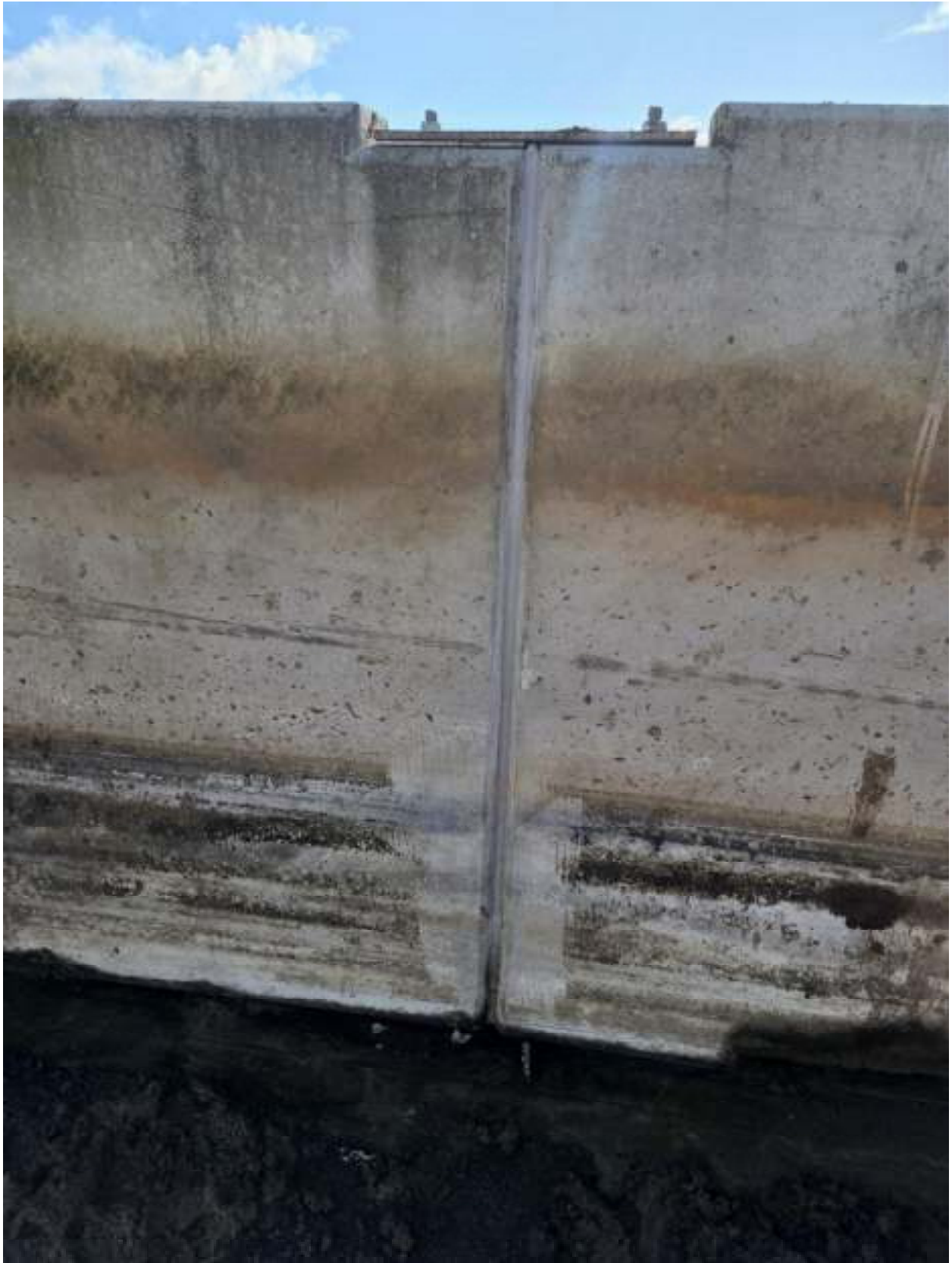
Figure 46 Panel joints of south sludge bed with repaired sealant.
