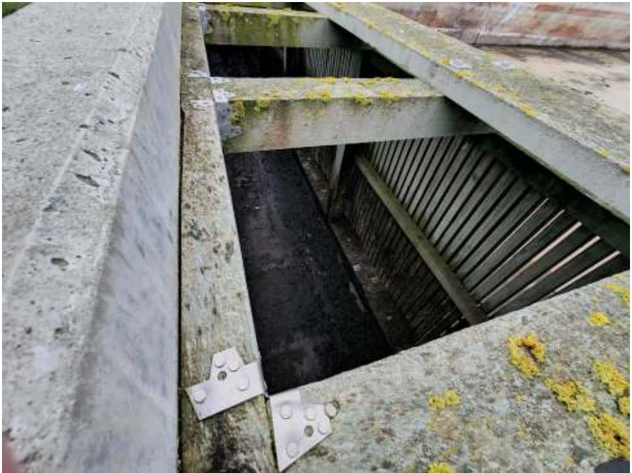
Figure 6 Interior of weeping wall structure.
