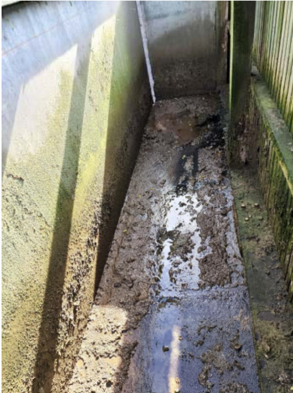
Figure 29 Panel joints of north sludge bed with repaired sealant.
