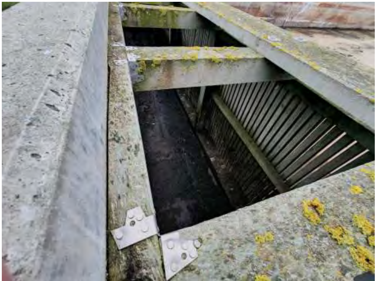
Figure 6 Interior of weeping wall structure.
