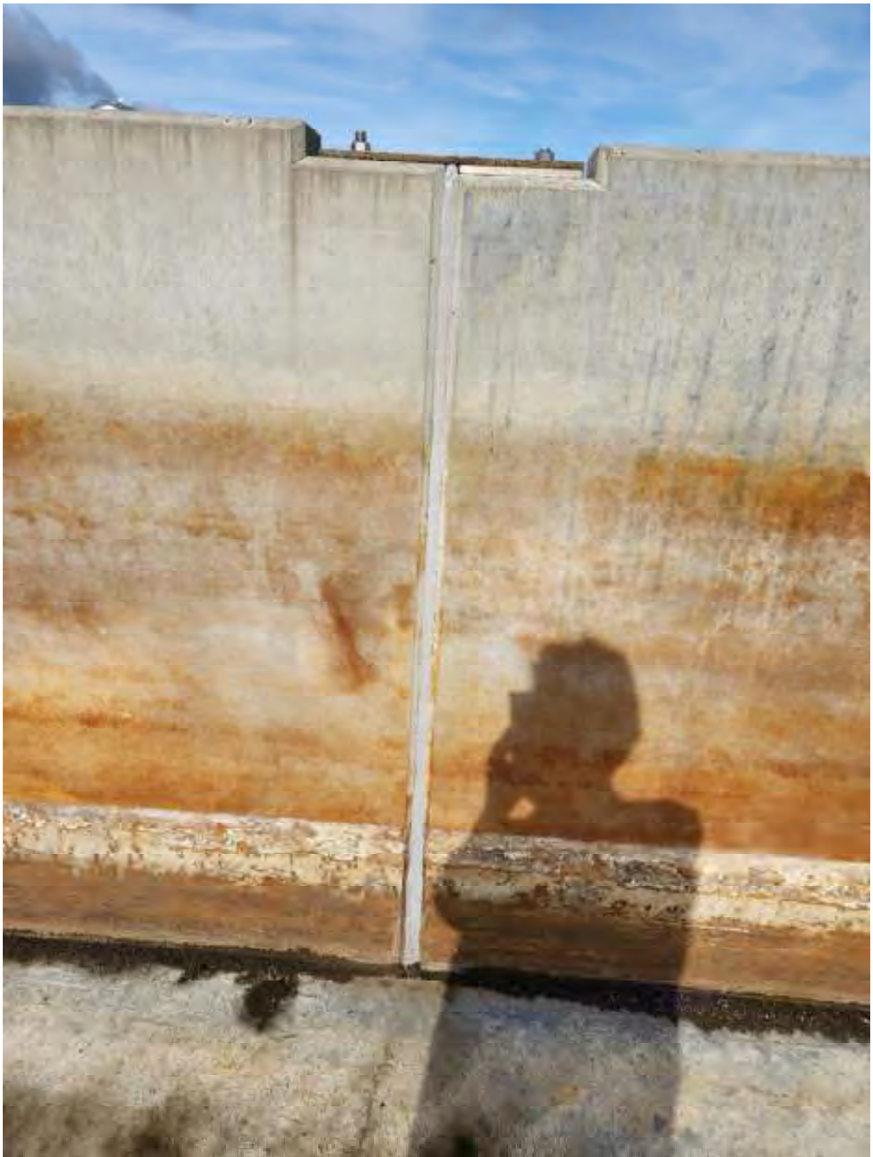
Figure 28 Panel joints of north sludge bed with repaired sealant.
