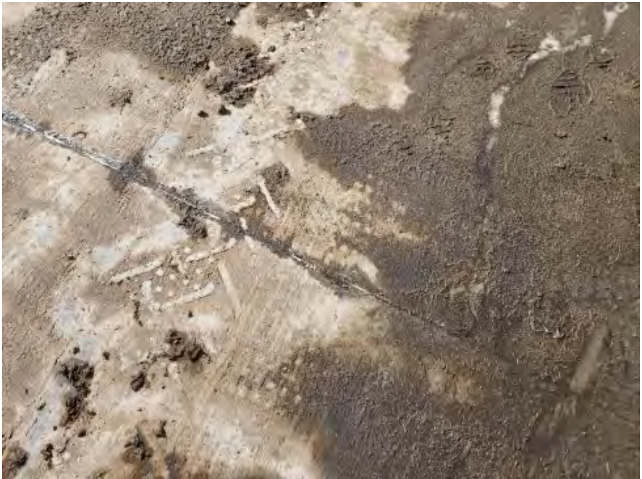
Figure 39 Floor joint of south sludge bed.
