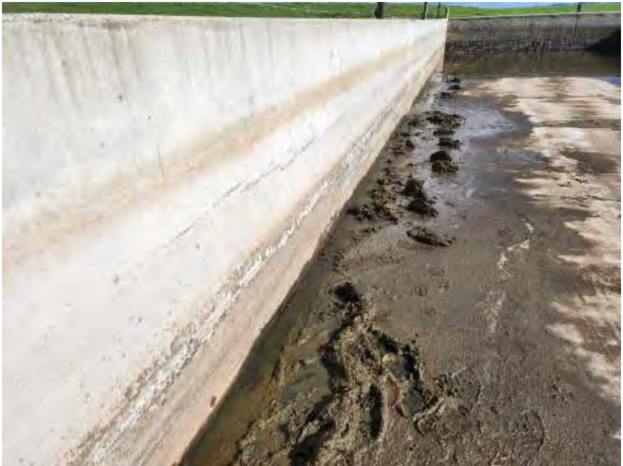
Figure 36 Edge join of south sludge bed.
