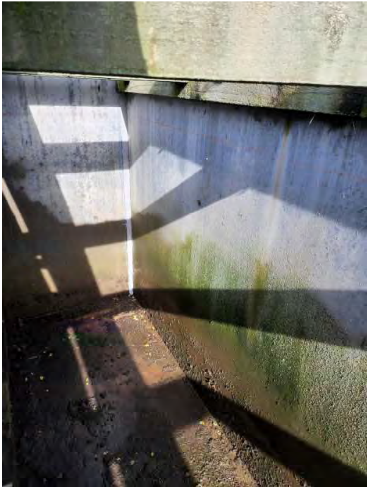
Figure 32 Panel joints of north sludge bed with repaired sealant.
