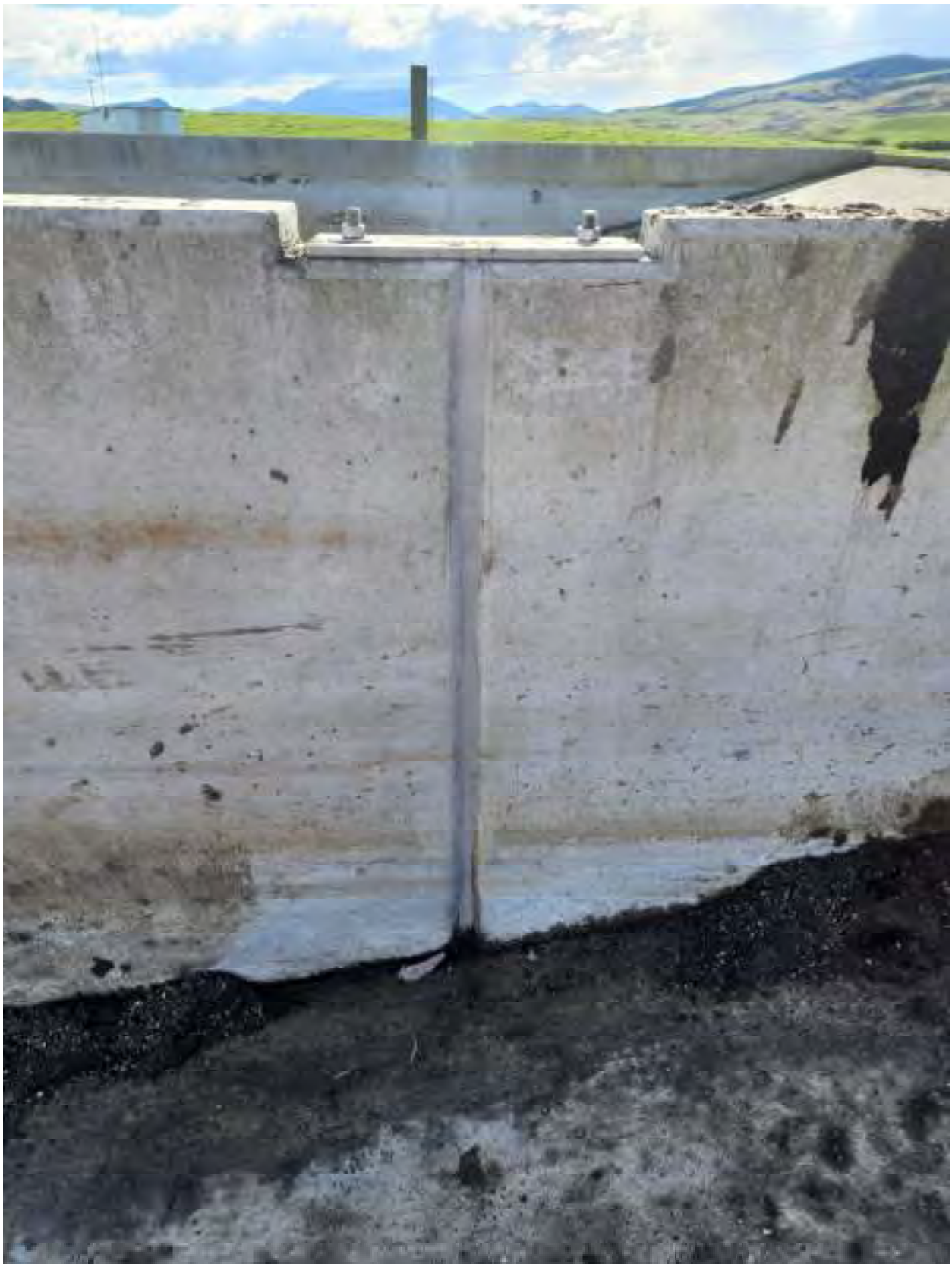
Figure 34 Panel joints of south sludge bed with repaired sealant.
