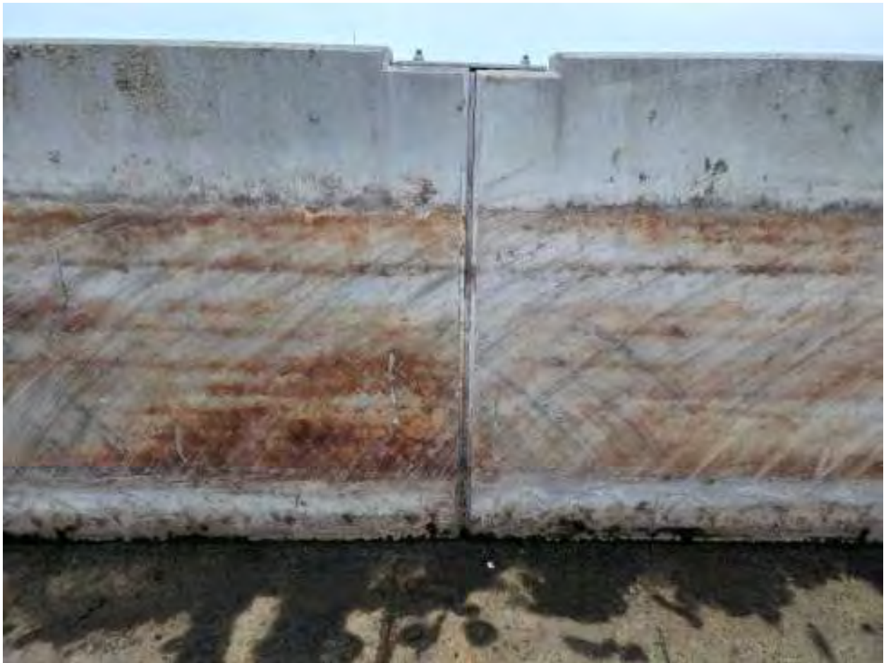
Figure 12 Panel joints of north sludge bed.
