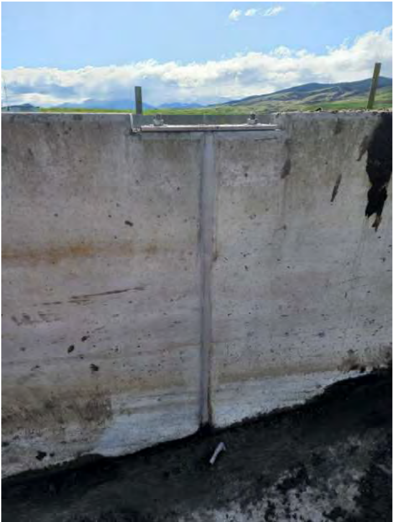
Figure 44 Panel joints of south sludge bed with repaired sealant.
