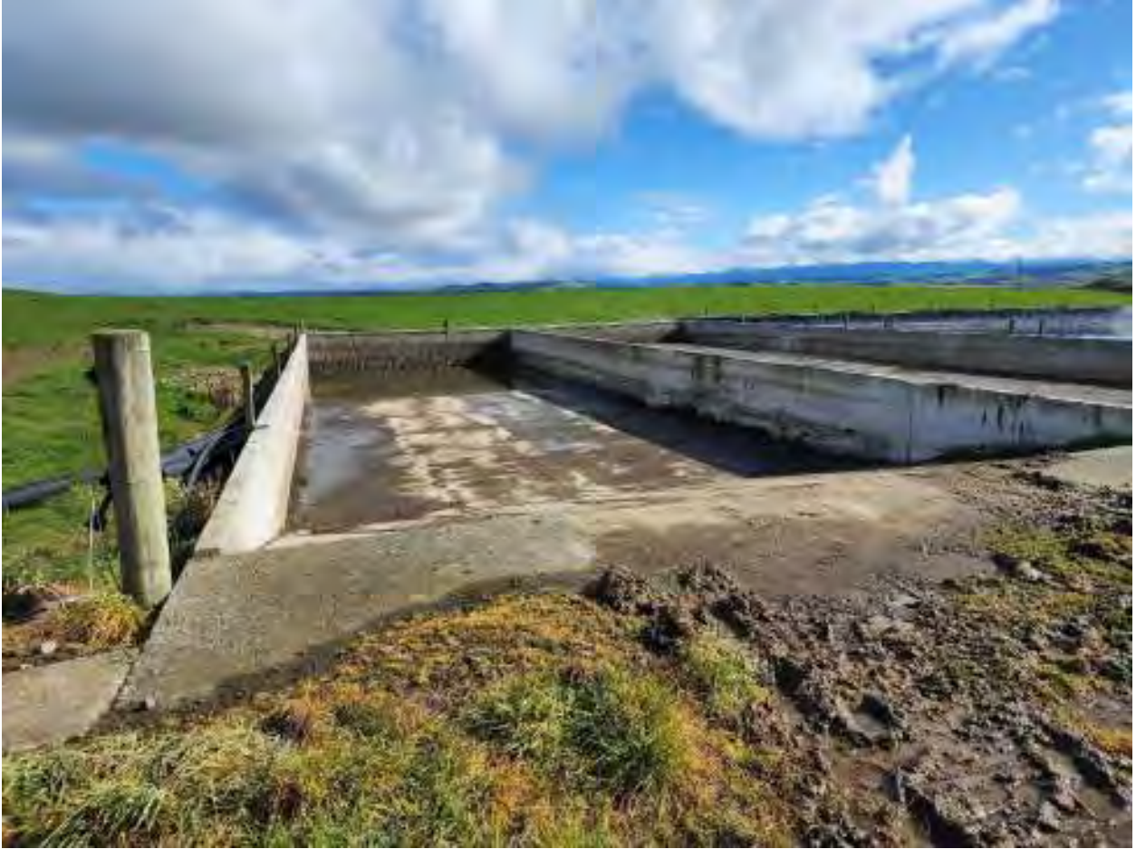
Figure 33 Interior of south sludge bed.
