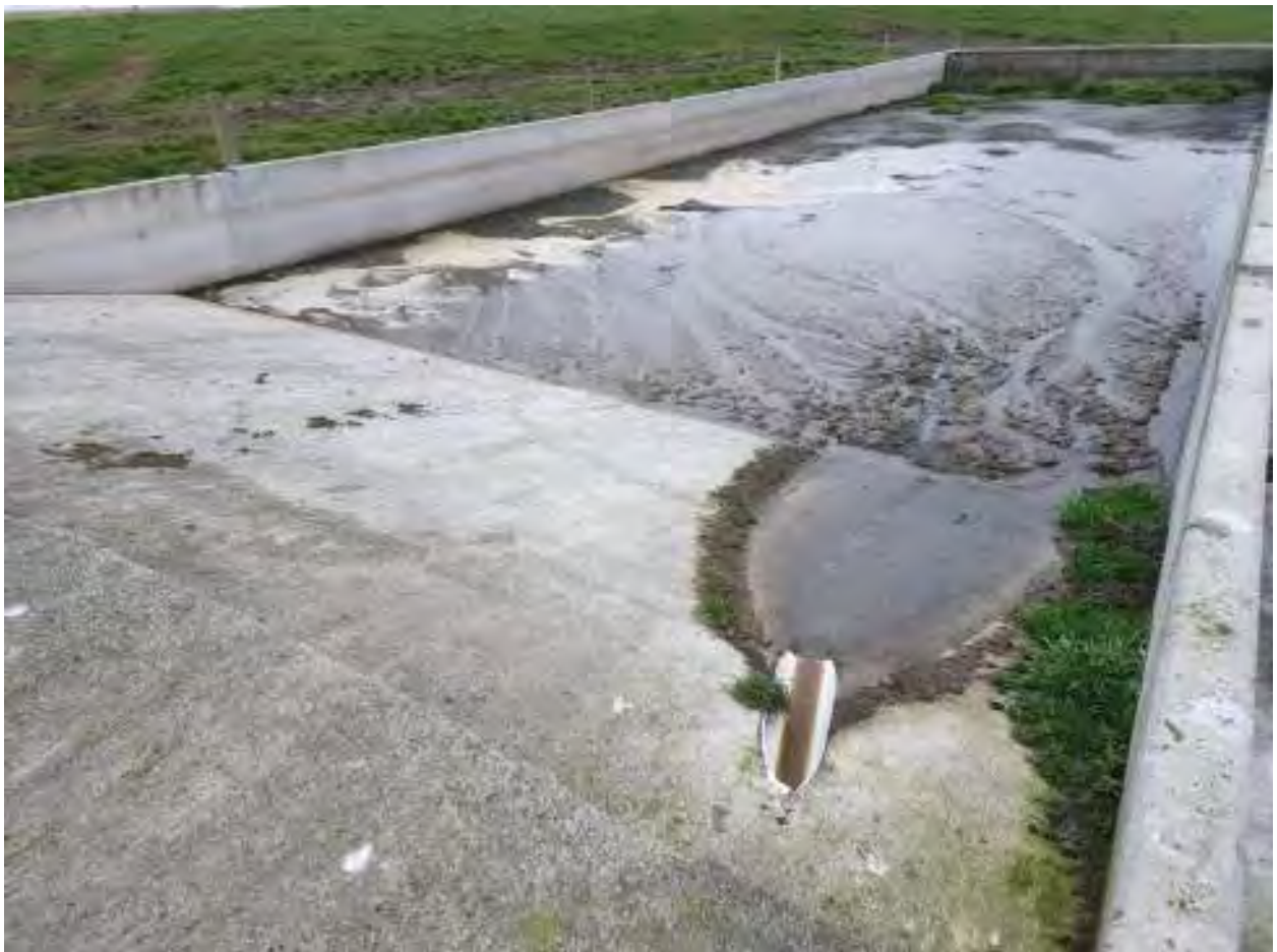
Figure 9 South sludge bed.
