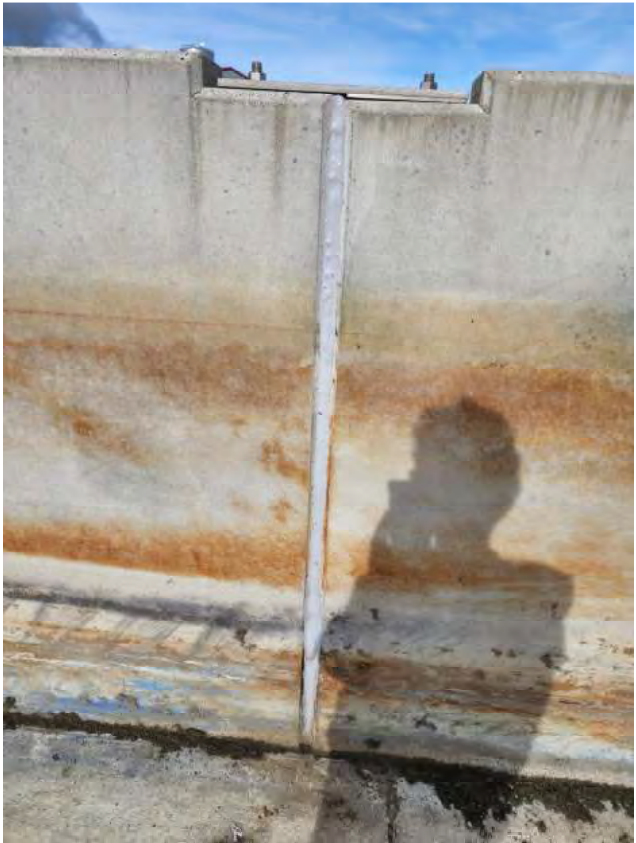
Figure 25 Panel joints of north sludge bed with repaired sealant.
