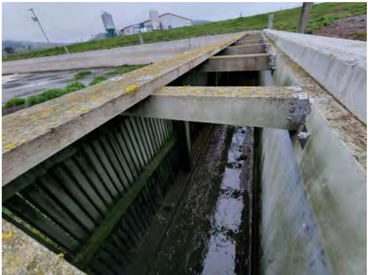
Figure 7 Interior of weeping wall structure.
