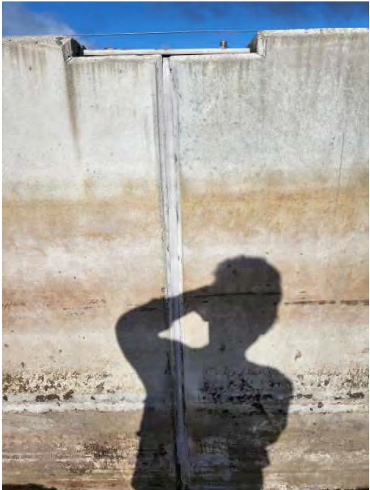
Figure 41 Panel joints of south sludge bed with repaired sealant.
