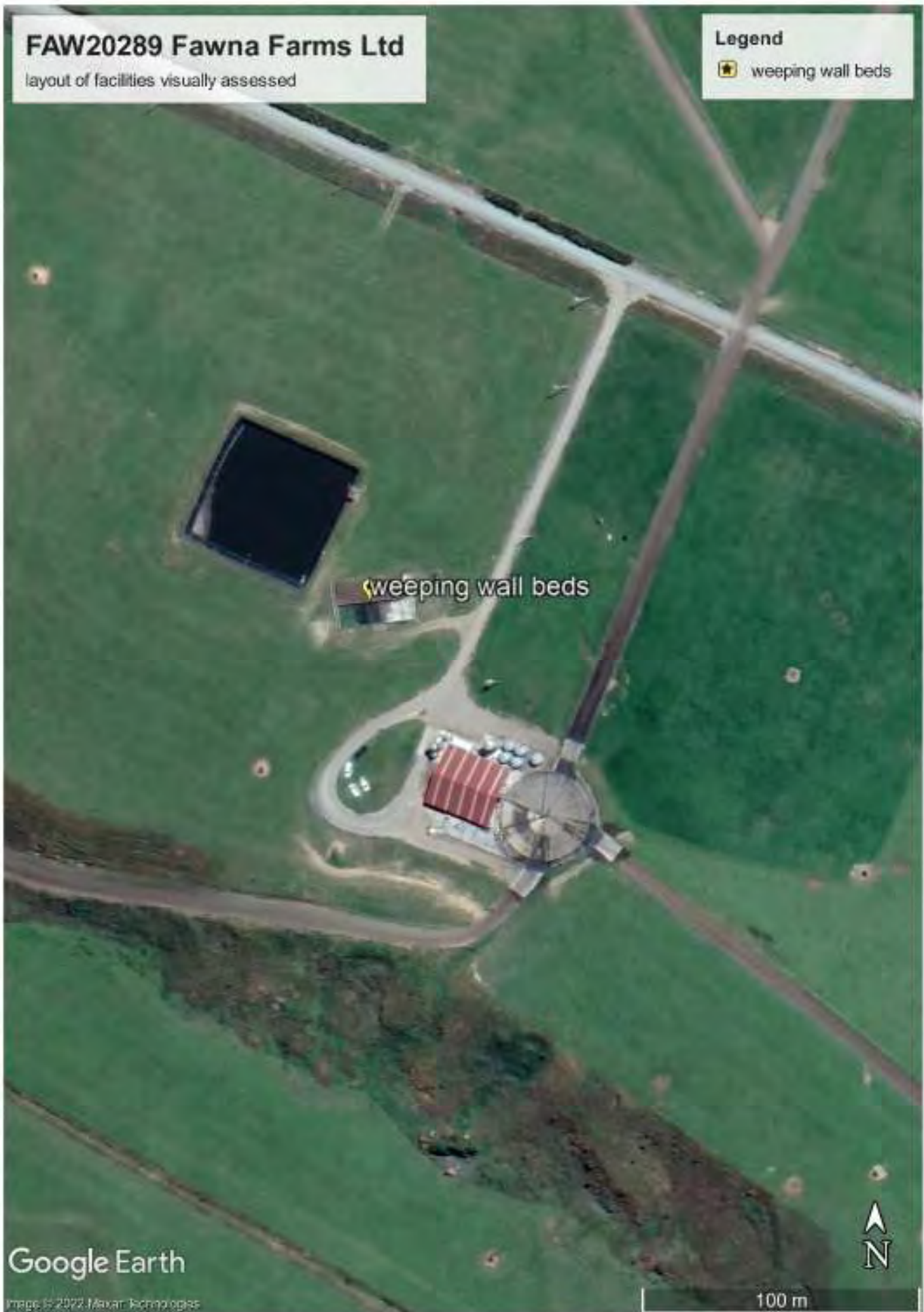
Figure 1 Layout of the facilities visually assessed.
