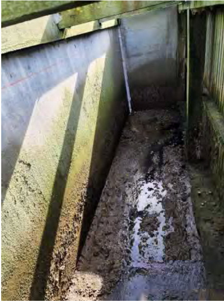
Figure 30 Panel joints of north sludge bed with repaired sealant.
