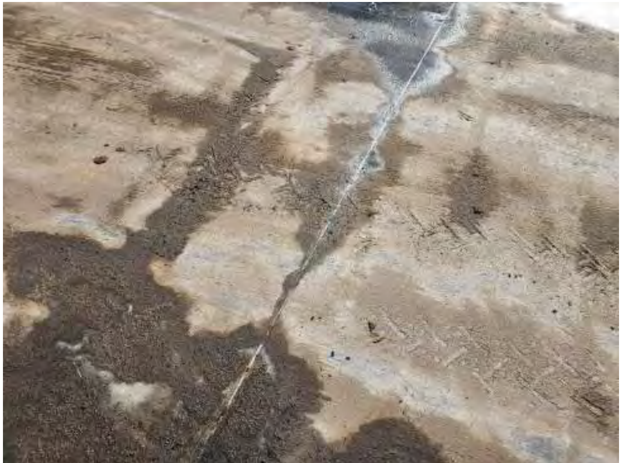
Figure 43 Edge joint of south sludge bed.
