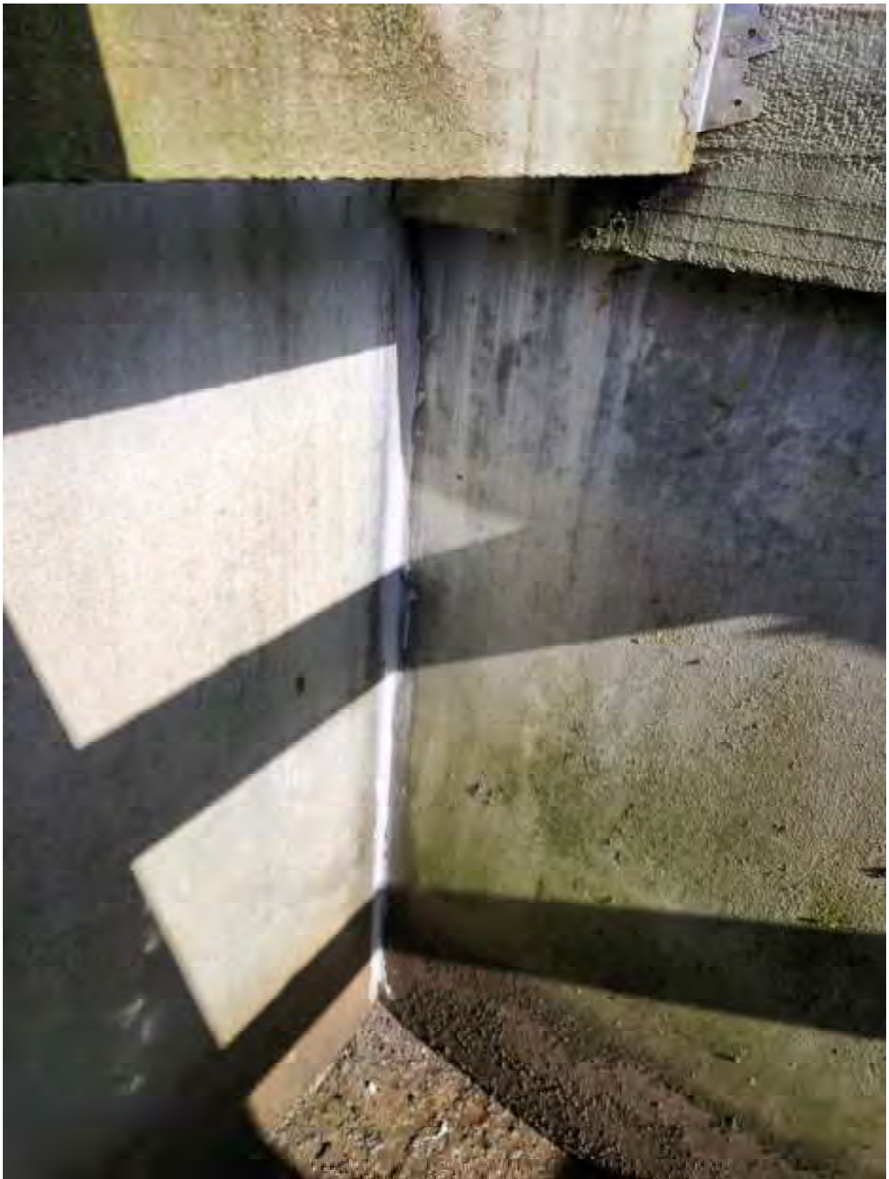
Figure 50 Panel joints of south sludge bed with repaired sealant.
