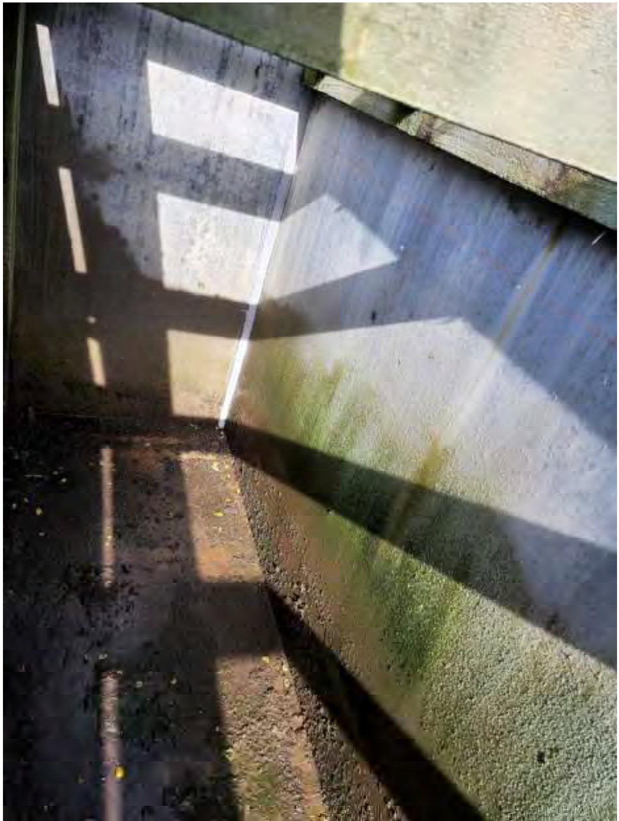
Figure 31 Panel joints of north sludge bed with repaired sealant.
