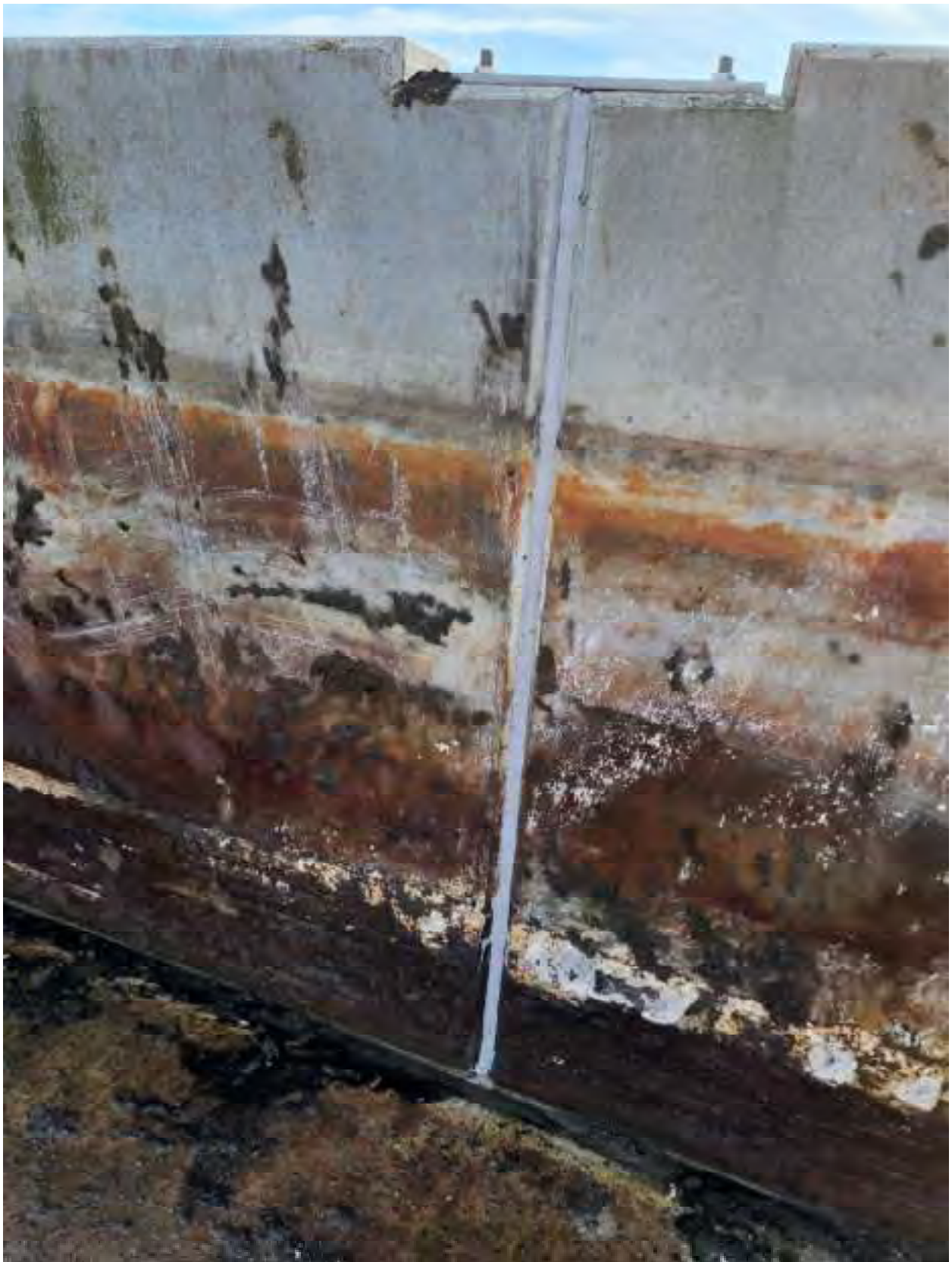
Figure 26 Panel joints of north sludge bed with repaired sealant.
