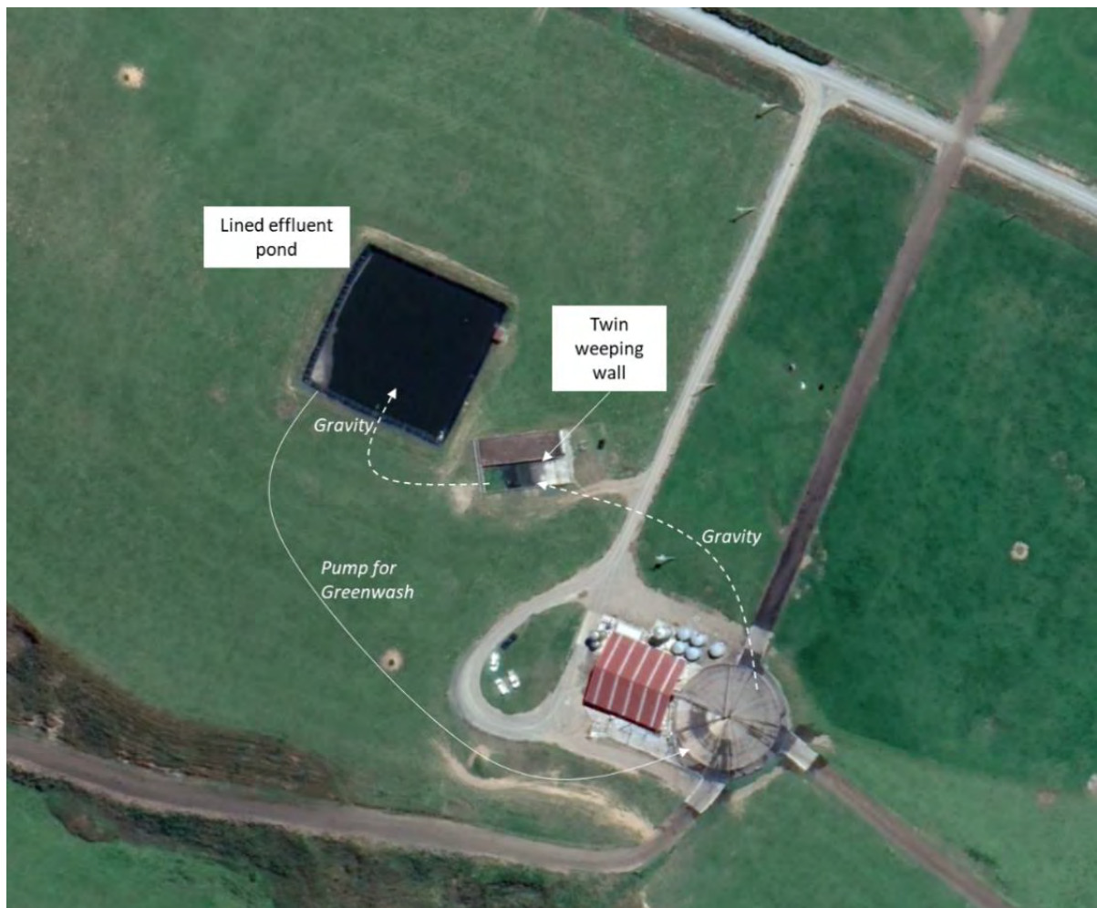
Figure 3: Effluent system overview.
