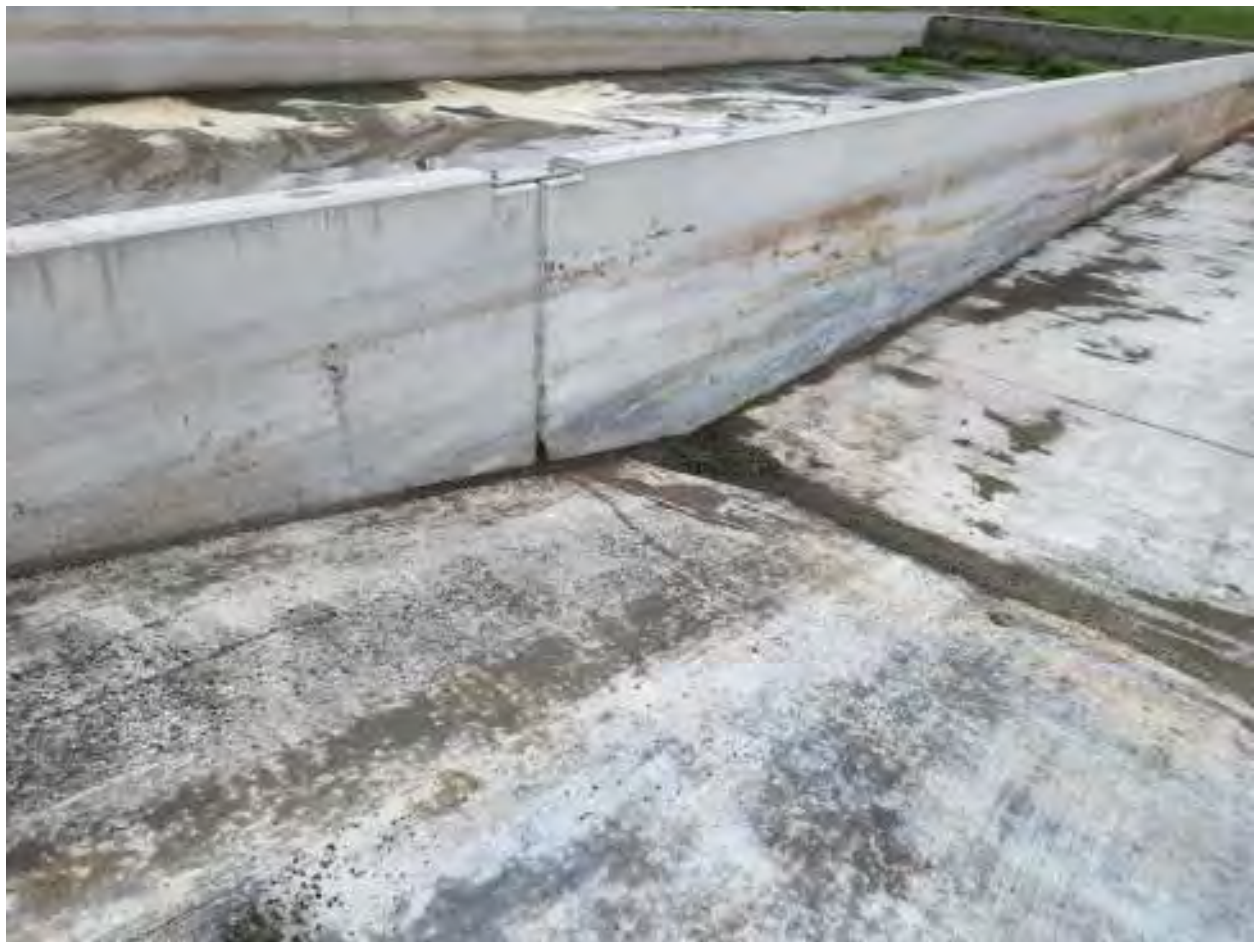
Figure 10 Interior of north sludge bed.
