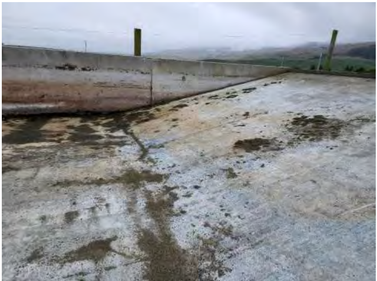
Figure 11 Interior of north sludge bed.
