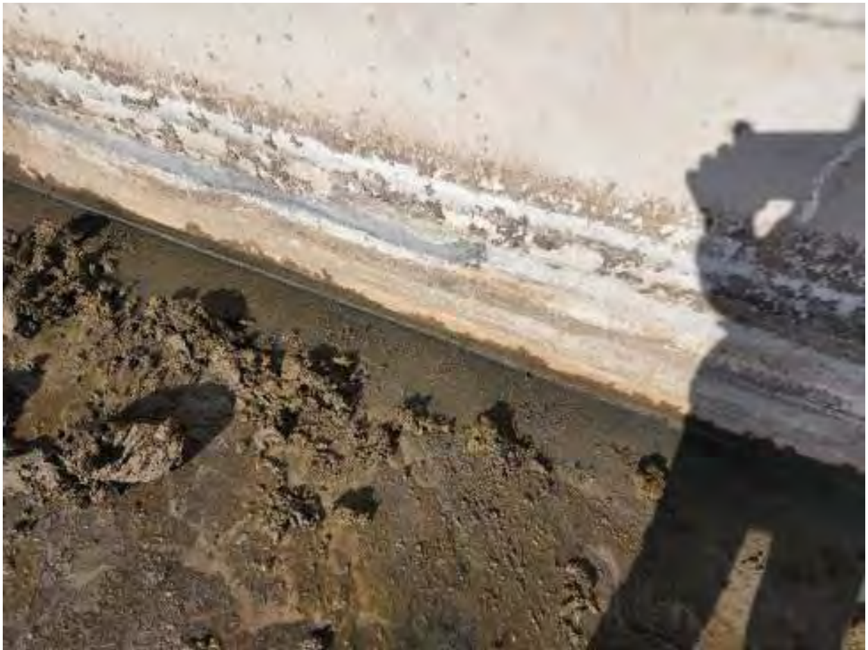
Figure 38 Edge joint of south sludge bed.
