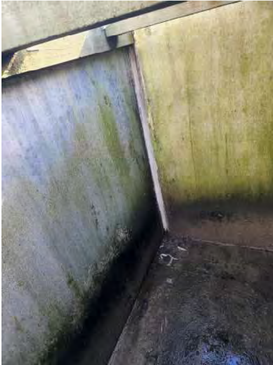
Figure 51 Panel joints of south sludge bed with repaired sealant.
