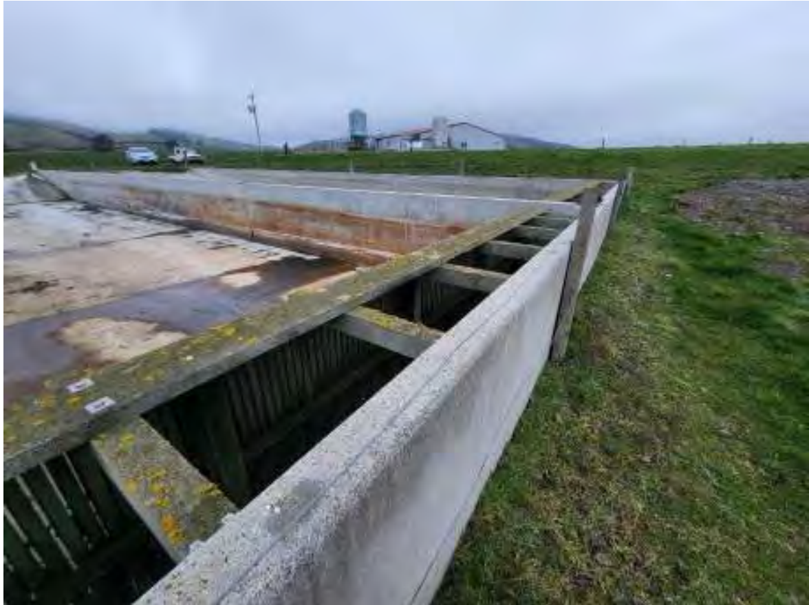
Figure 2 Weeping wall structure and exterior of facility.
