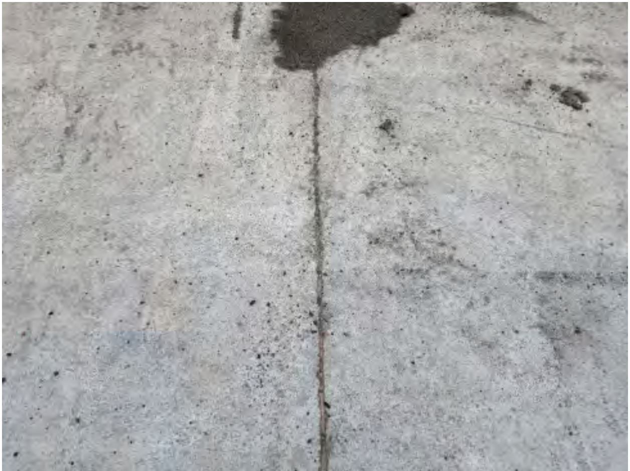
Figure 14 Floor joints of north sludge bed.
