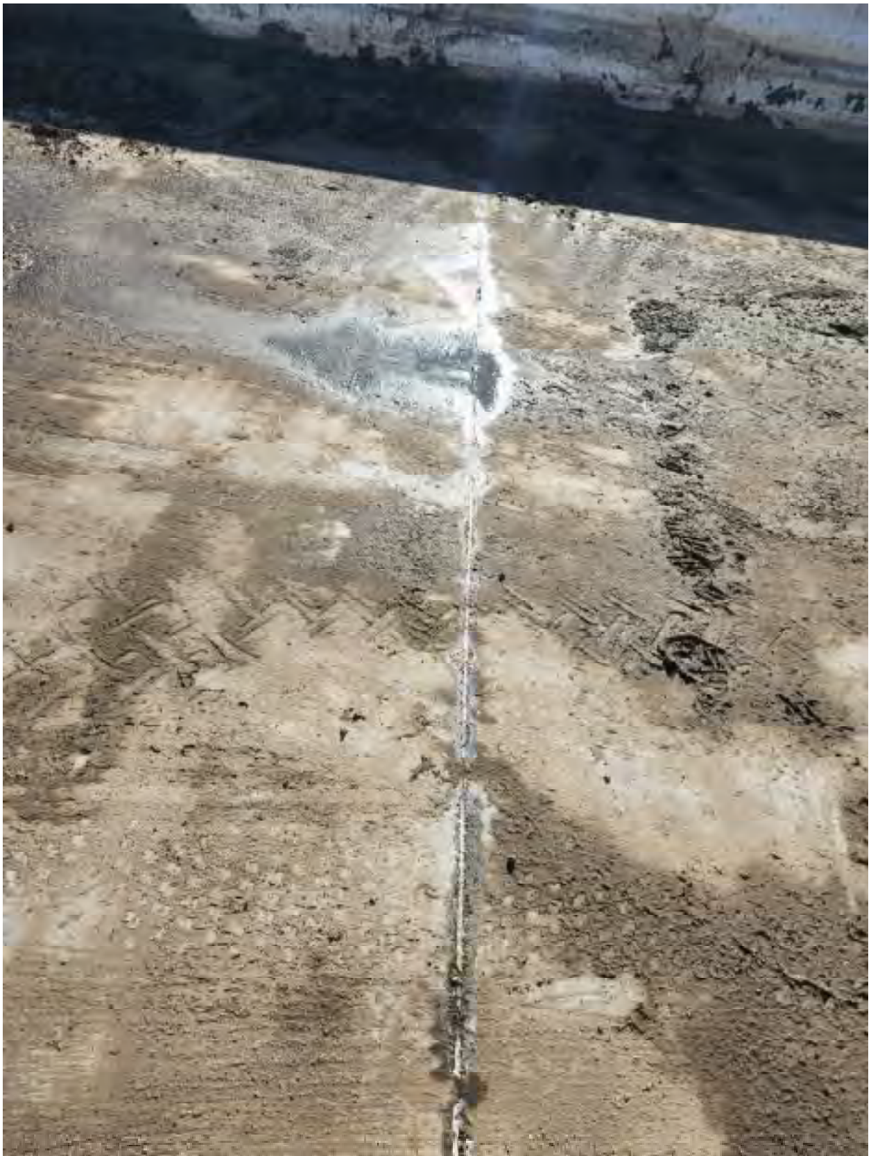
Figure 40 Floor joint of south sludge bed.
