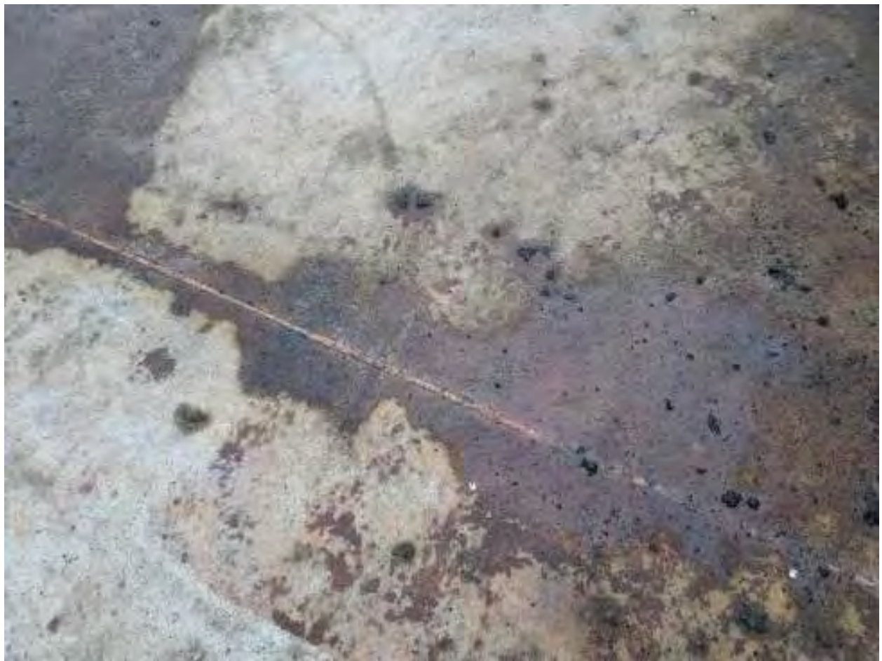
Figure 16 Floor joints of north sludge bed.
