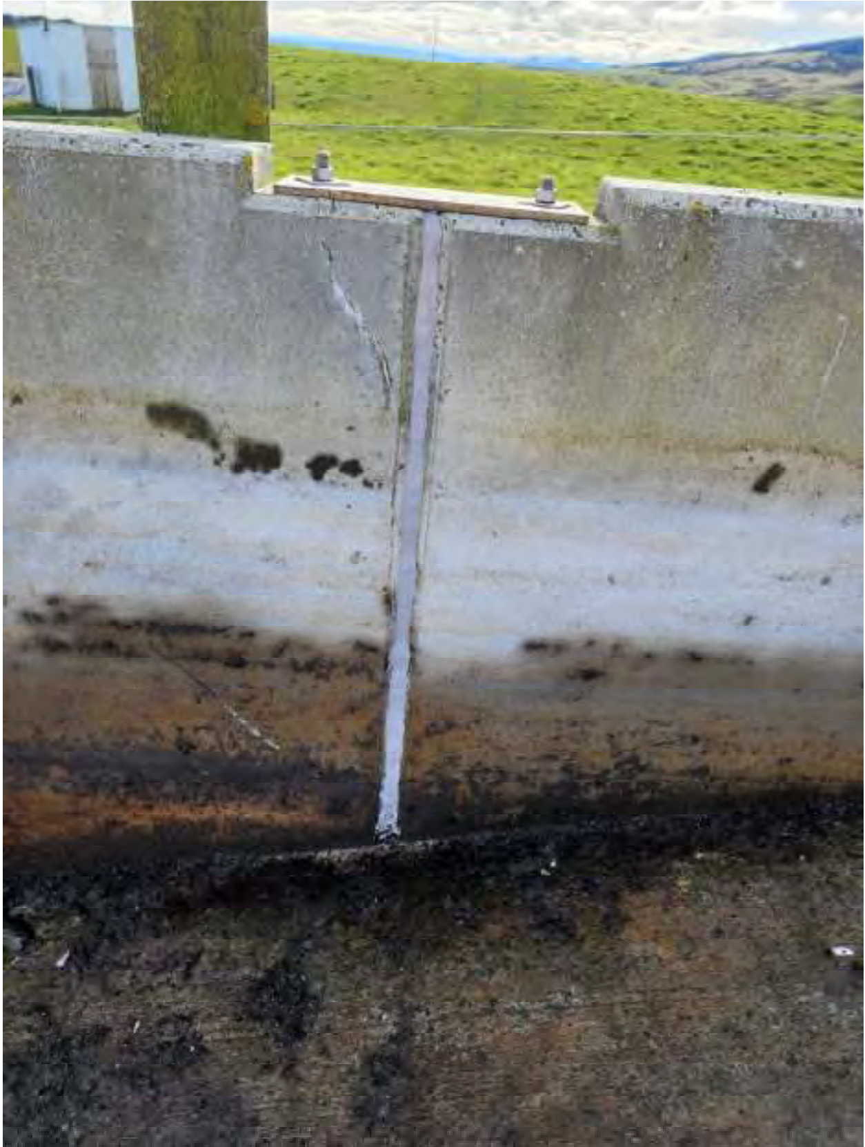
Figure 21 Panel joints of north sludge bed with repaired sealant.
