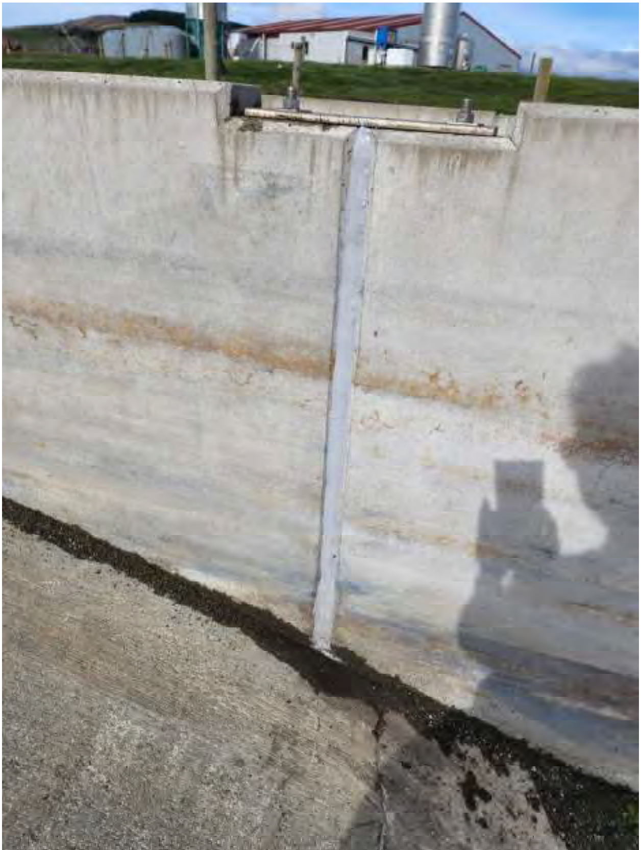
Figure 22 Panel joints of north sludge bed with repaired sealant.
