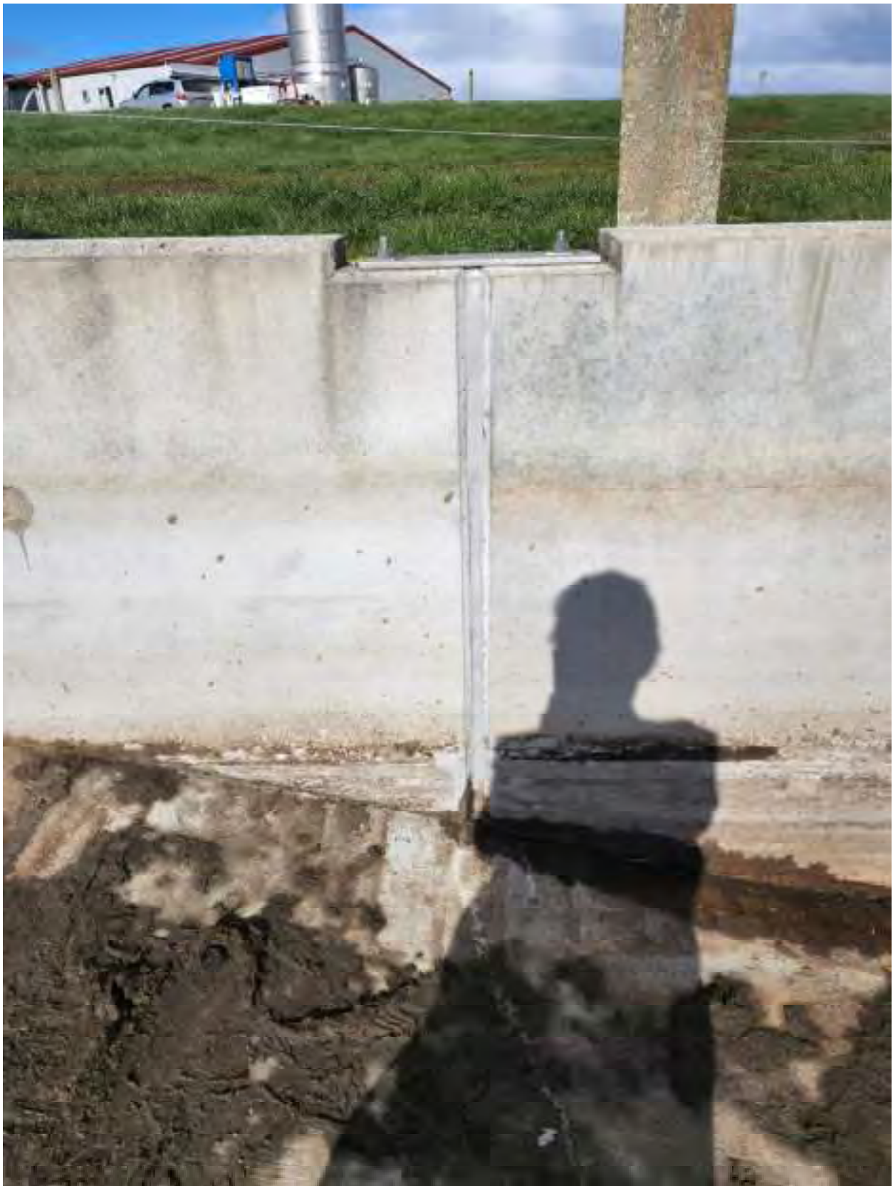
Figure 35 Panel joints of south sludge bed with repaired sealant.
