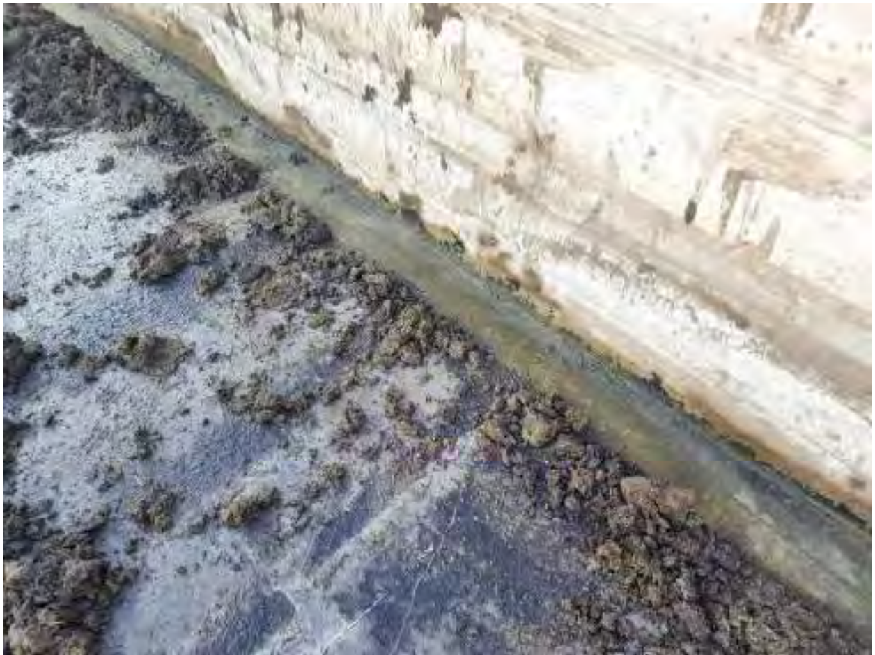
Figure 45 Edge joint of south sludge bed.
