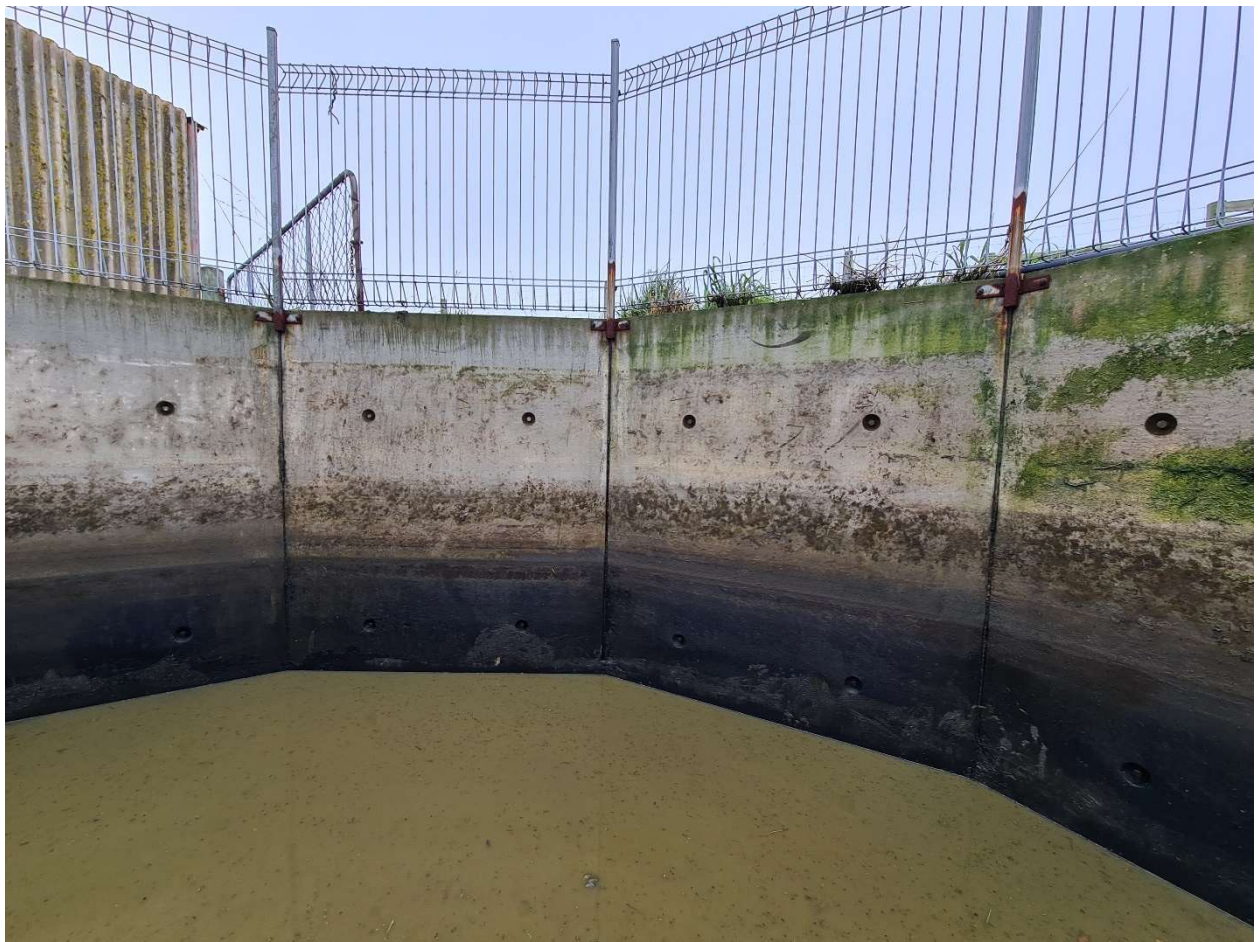
Figure 10 Interior panels of facility
