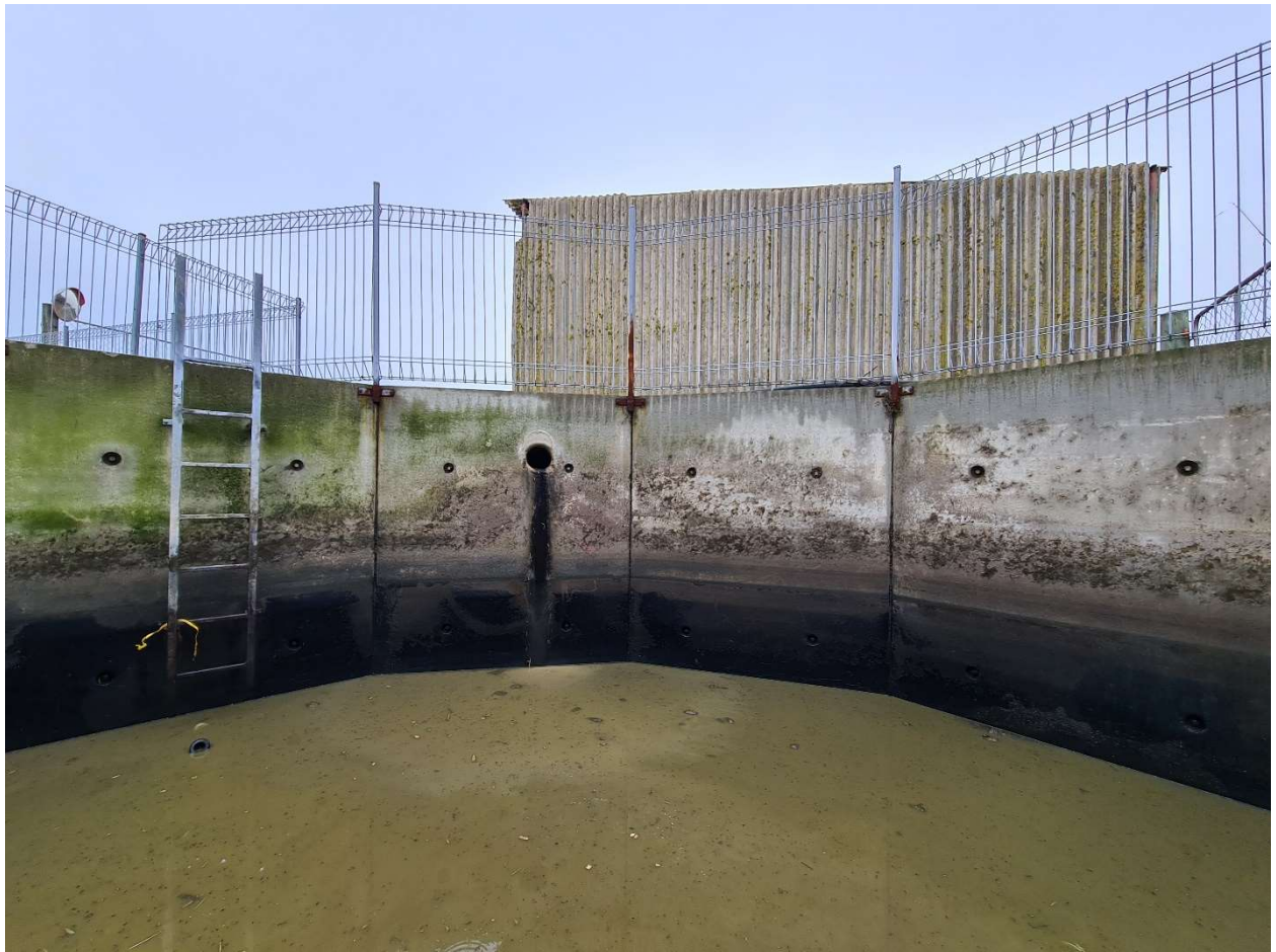
Figure 8 Interior panels of facility
