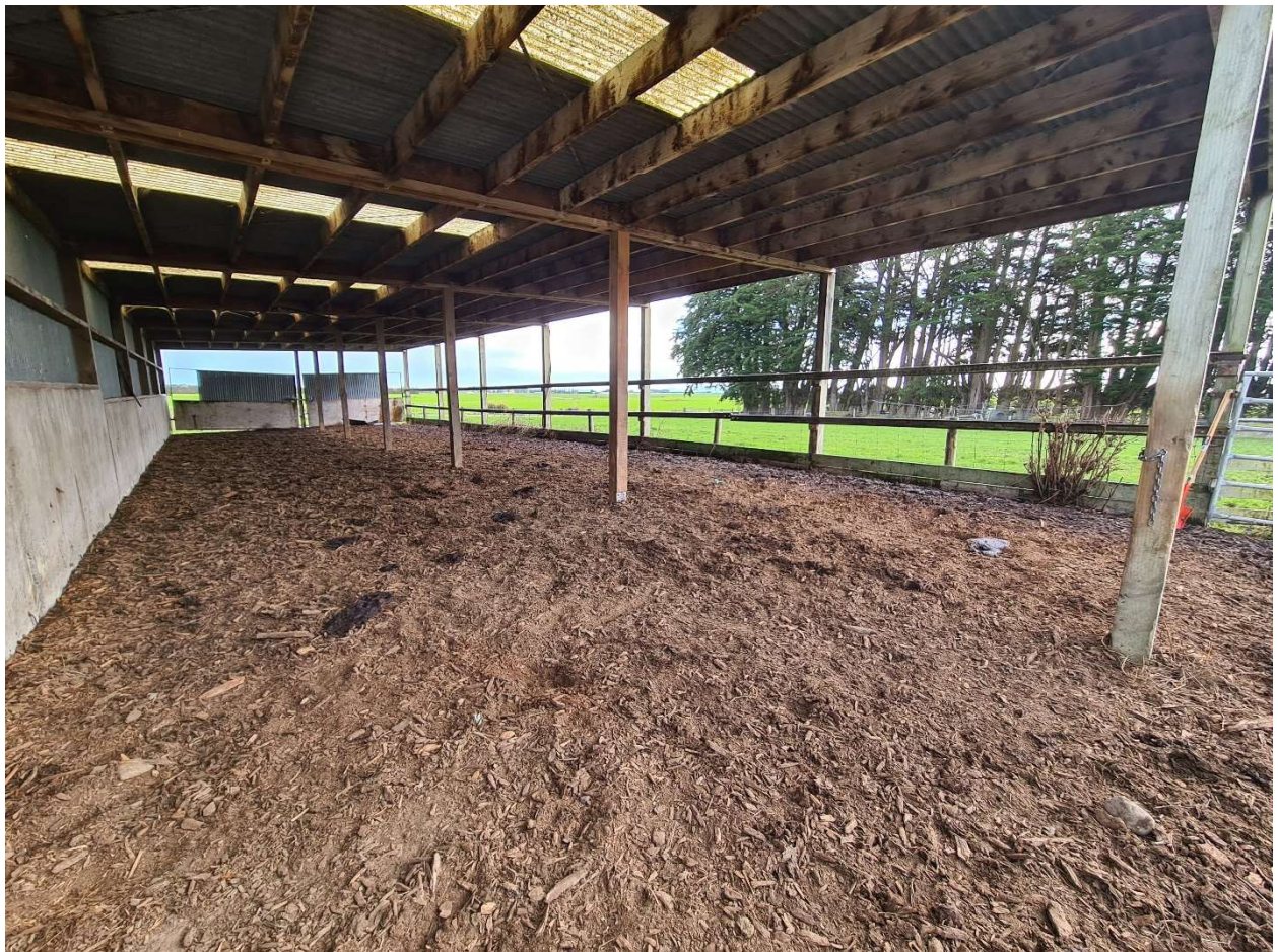
Figure 8 View of the roofed area of the facility looking north-west showing the roof and layer of woodchip across the facility.
