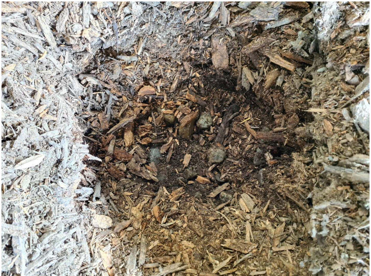
Figure 6 Pit dug in the south half of the roofed area showing layer of woodchip on top of a compacted rock base.
