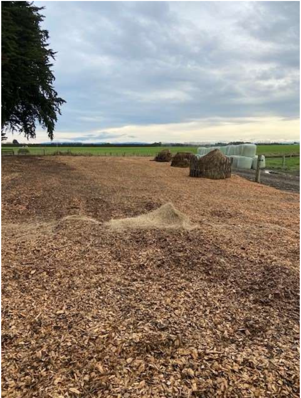
Figure 31 View of facility looking west showing the layer of woodchip spread across the base of the facility (photo supplied by consent holder).
