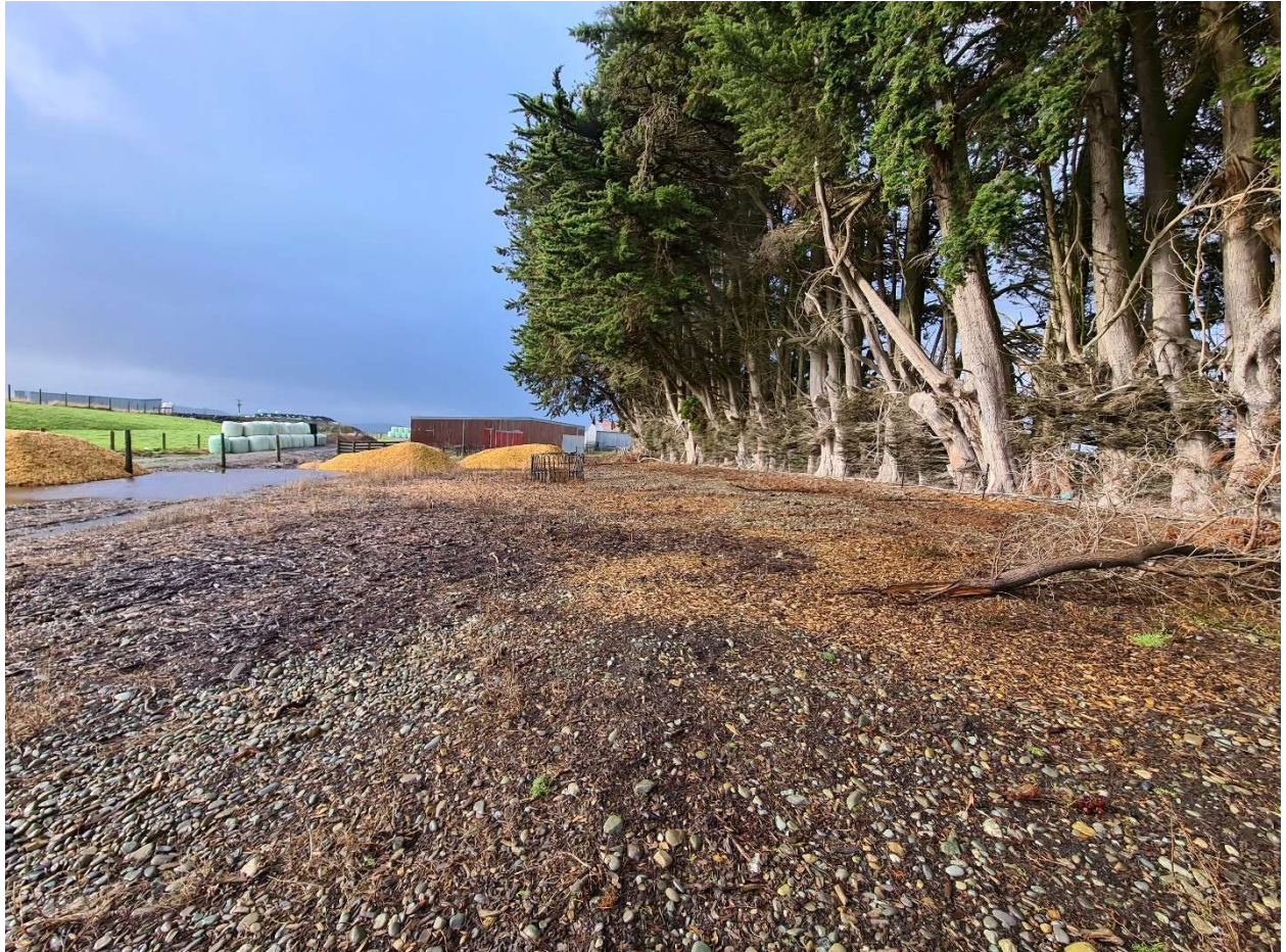
Figure 26 View of facility looking east showing woodchip ready to spread, the rock base and the hedgerow along the south edge of the facility.
