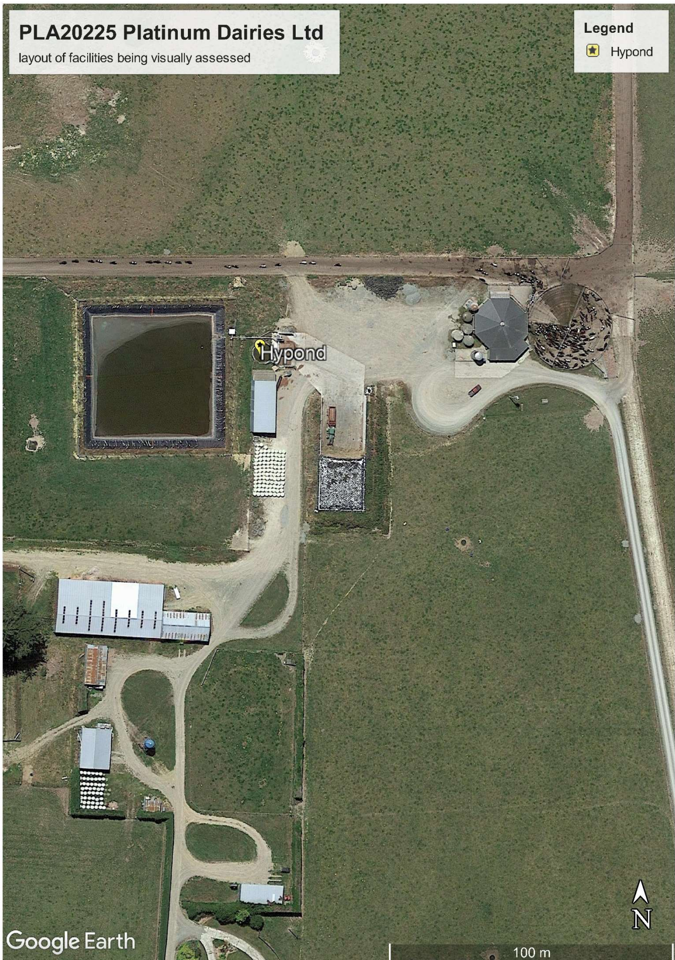
Figure 1 Layout of the facilities visually assessed.
