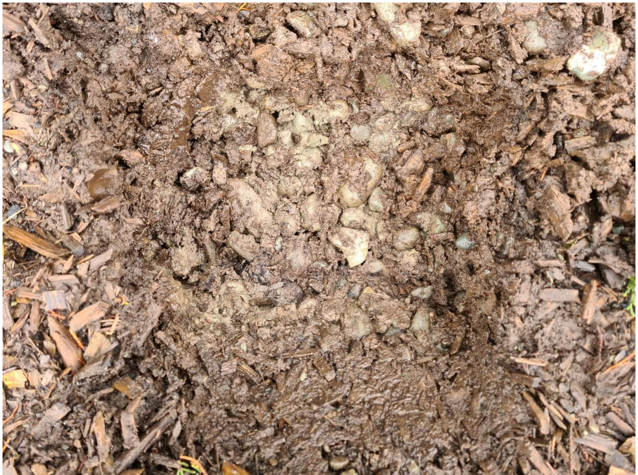
Figure 30 Pit dug showing compacted rock base.
