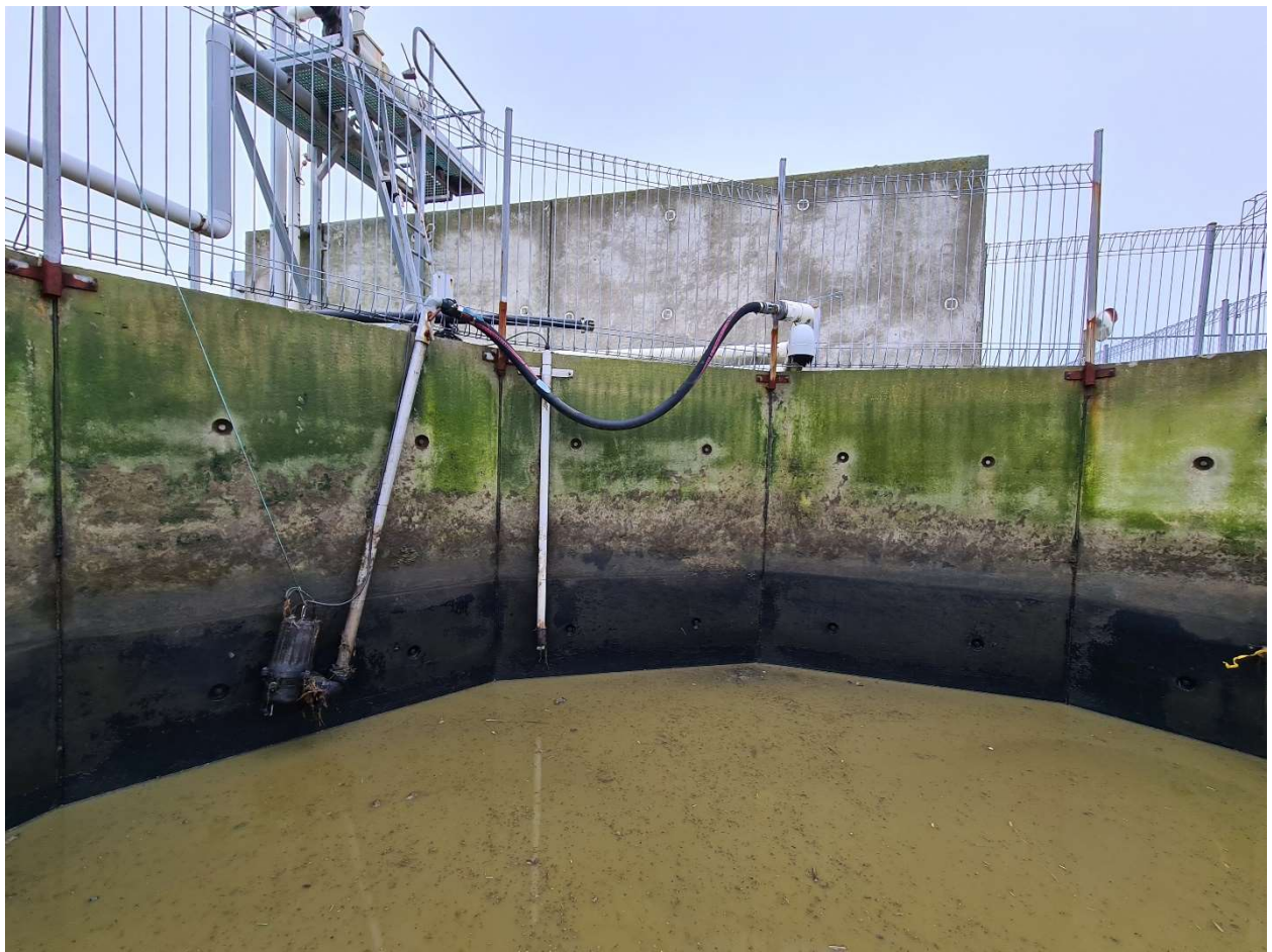
Figure 6 Interior panels of facility effluent pump, and float switch
