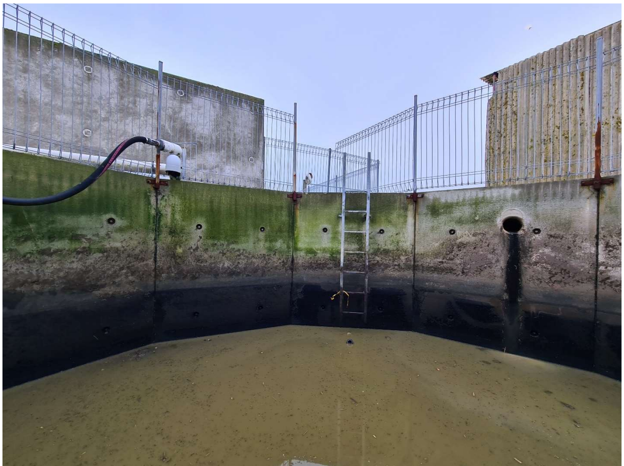
Figure 7 Interior panels of facility
