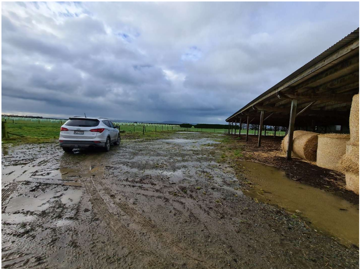
Figure 23 View of the uncovered area of the facility showing the lane material which was used to construct the base of the uncovered area.
