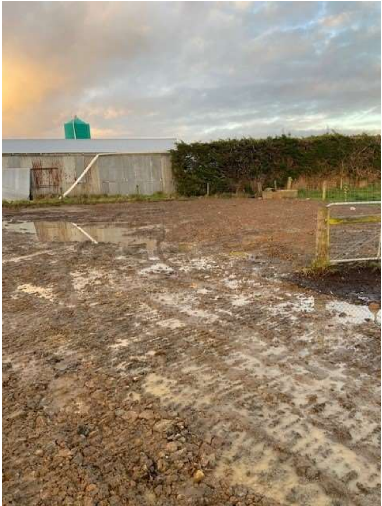
Figure 13 View of the compacted rock base of uncovered area looking east (photo supplied by consent holder).
