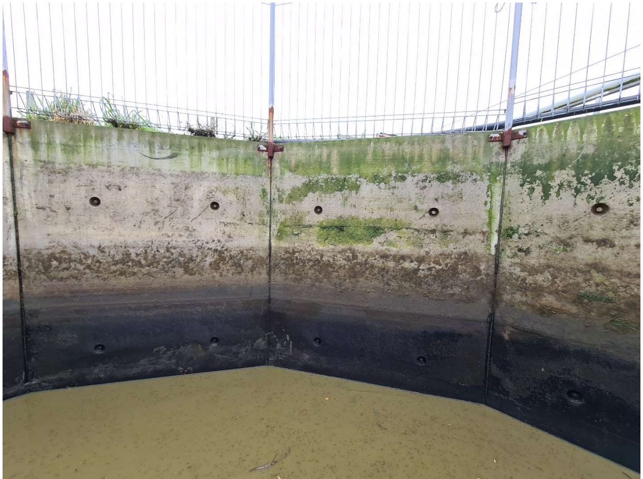
Figure 11 Interior panels of facility
