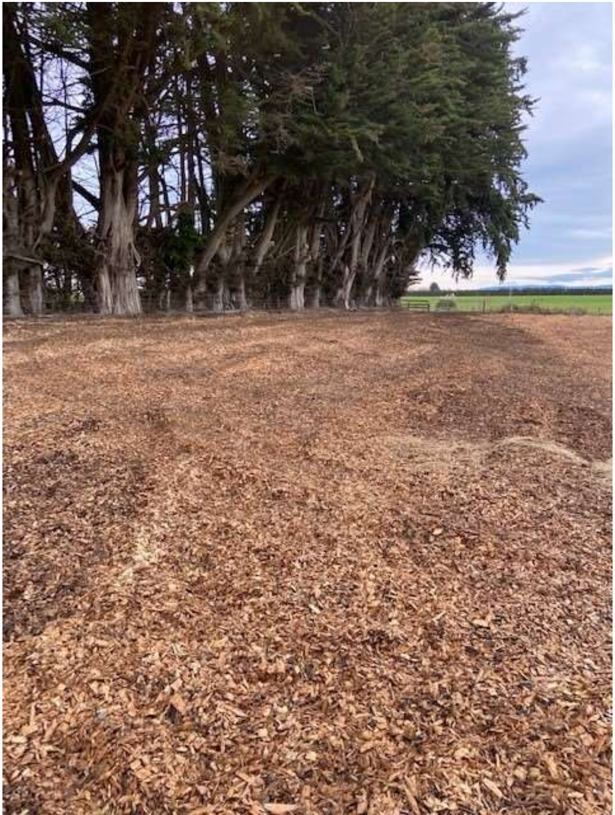
Figure 32 View of facility looking south-west showing the layer of woodchip spread across the base of the facility (photo supplied by consent holder).
