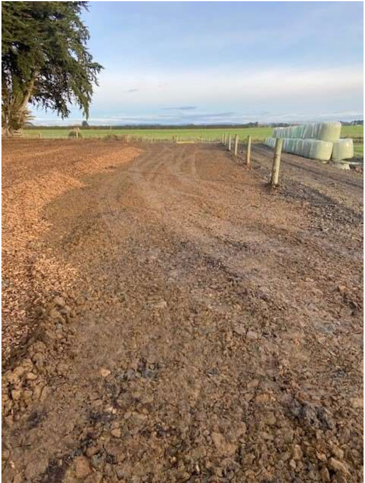
Figure 33 View of facility looing west showing where more compacted rock has been placed ready for woodchip to be spread (photo supplied by consent holder).
