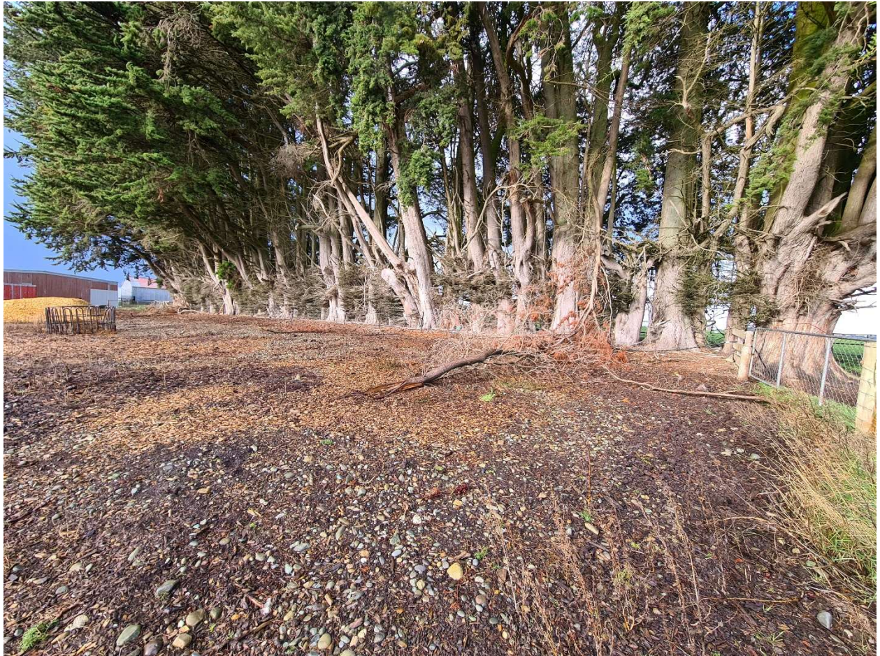
Figure 25 View of facility looking south-east showing the hedgerow and compacted rock base.
