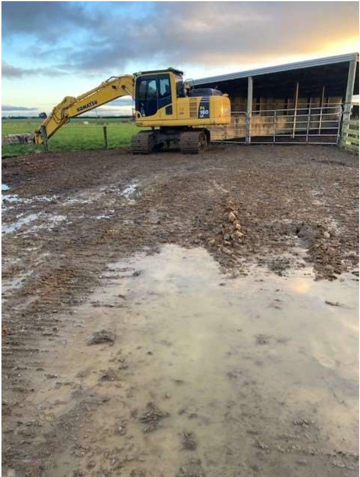
Figure 14 View of the compacted rock base of uncovered area looking south-west (photo supplied by consent holder).
