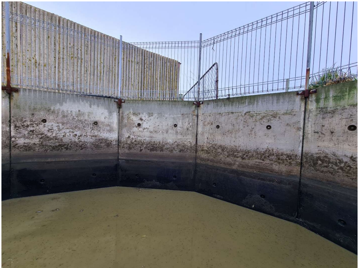
Figure 9 Interior panels of facility
