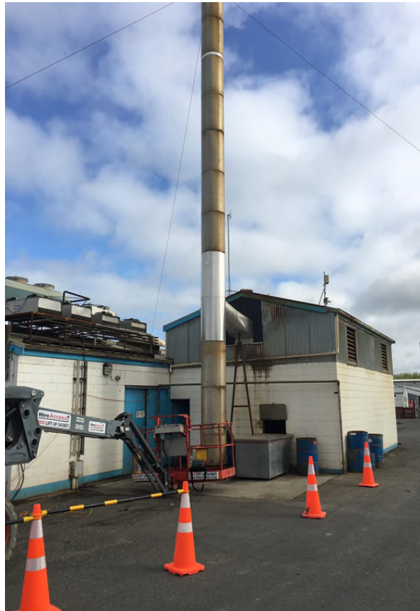
Figure 1. Photo of sampling location
