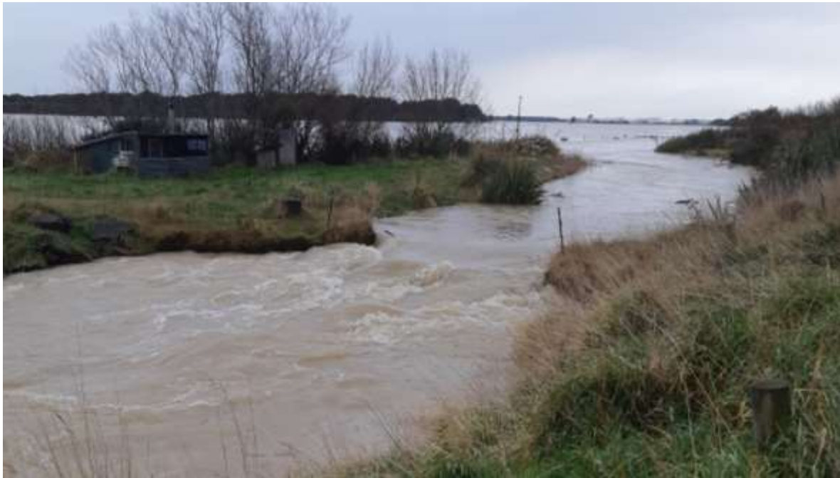
Figure 3 View of tidegates overflowing during flood
