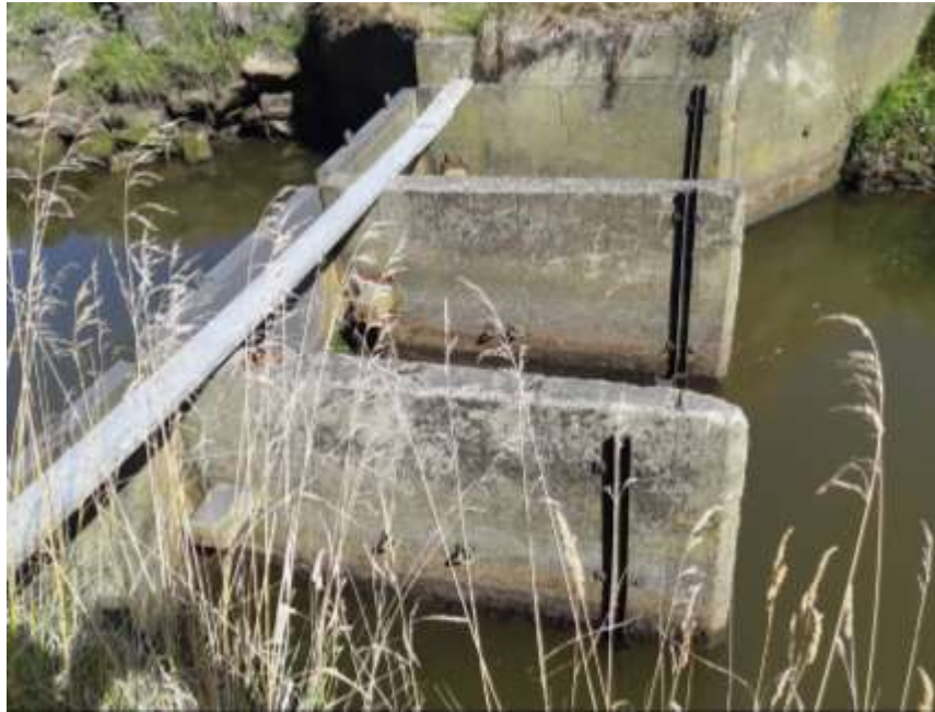
Figure 1 View from upstream side when closed
