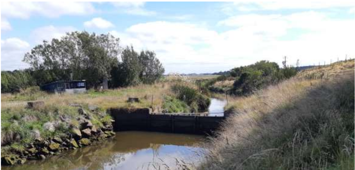
Figure 2 View of tidegates from downstream when closed
