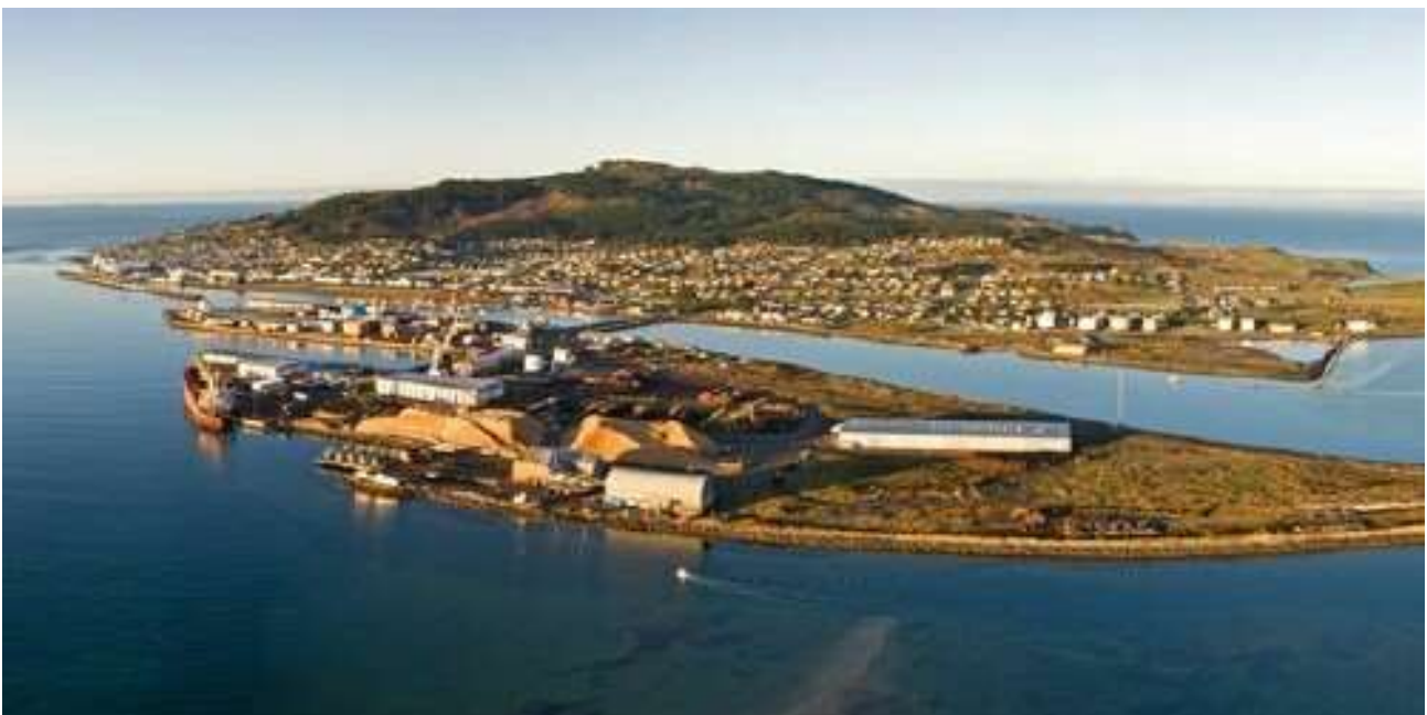
Figure 15 – Aerial photo looking towards the Bluff Township with Bluff Hill / Motupohue in the background
