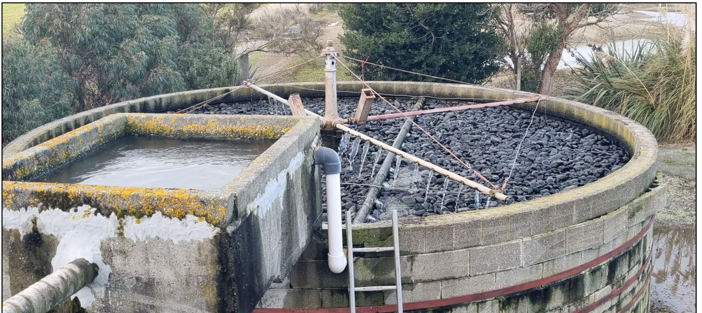
Figure 27 Trickling filter
