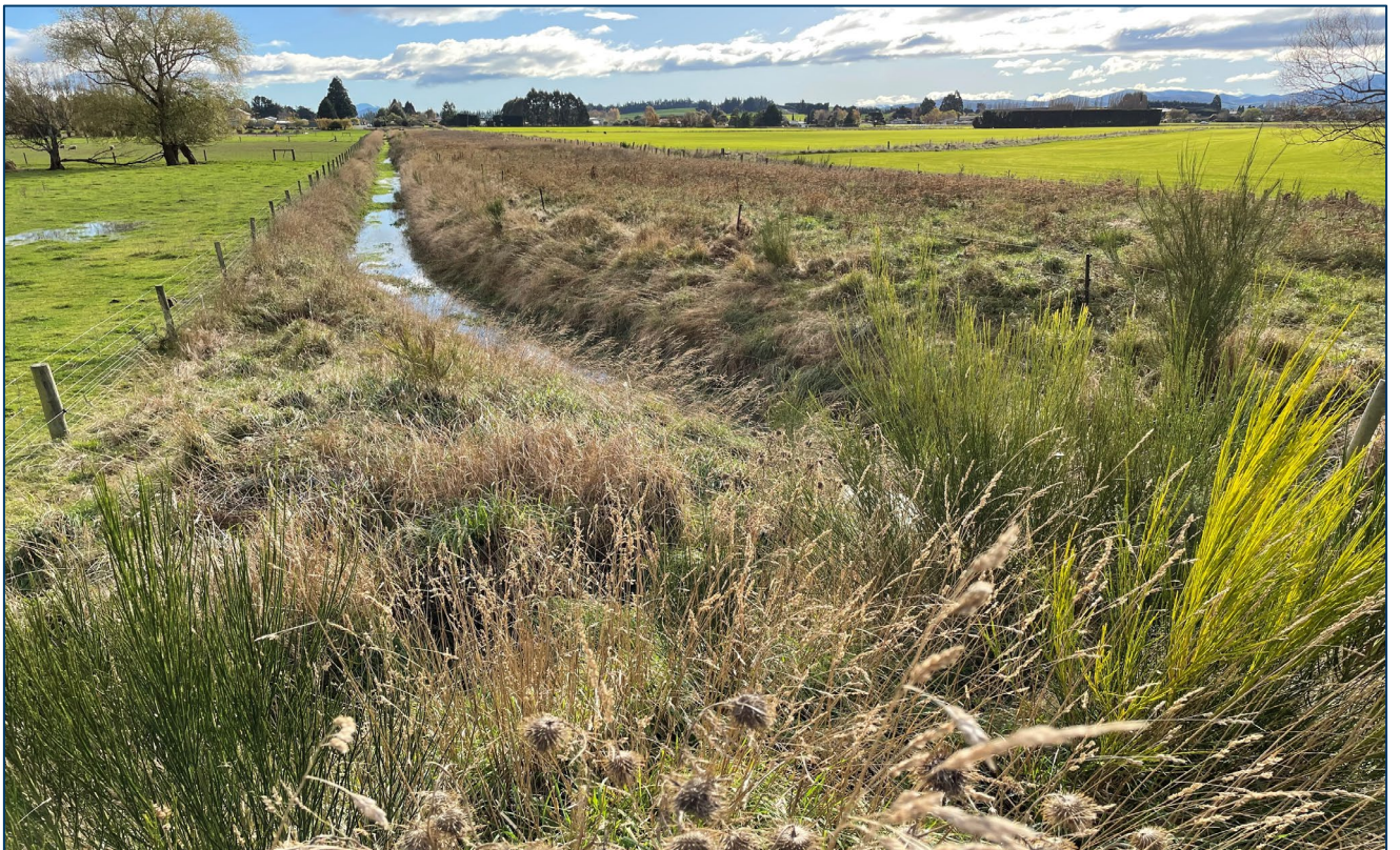
Figure 4 Drainage channel at bottom end prior to discharging into Longridge Stream
