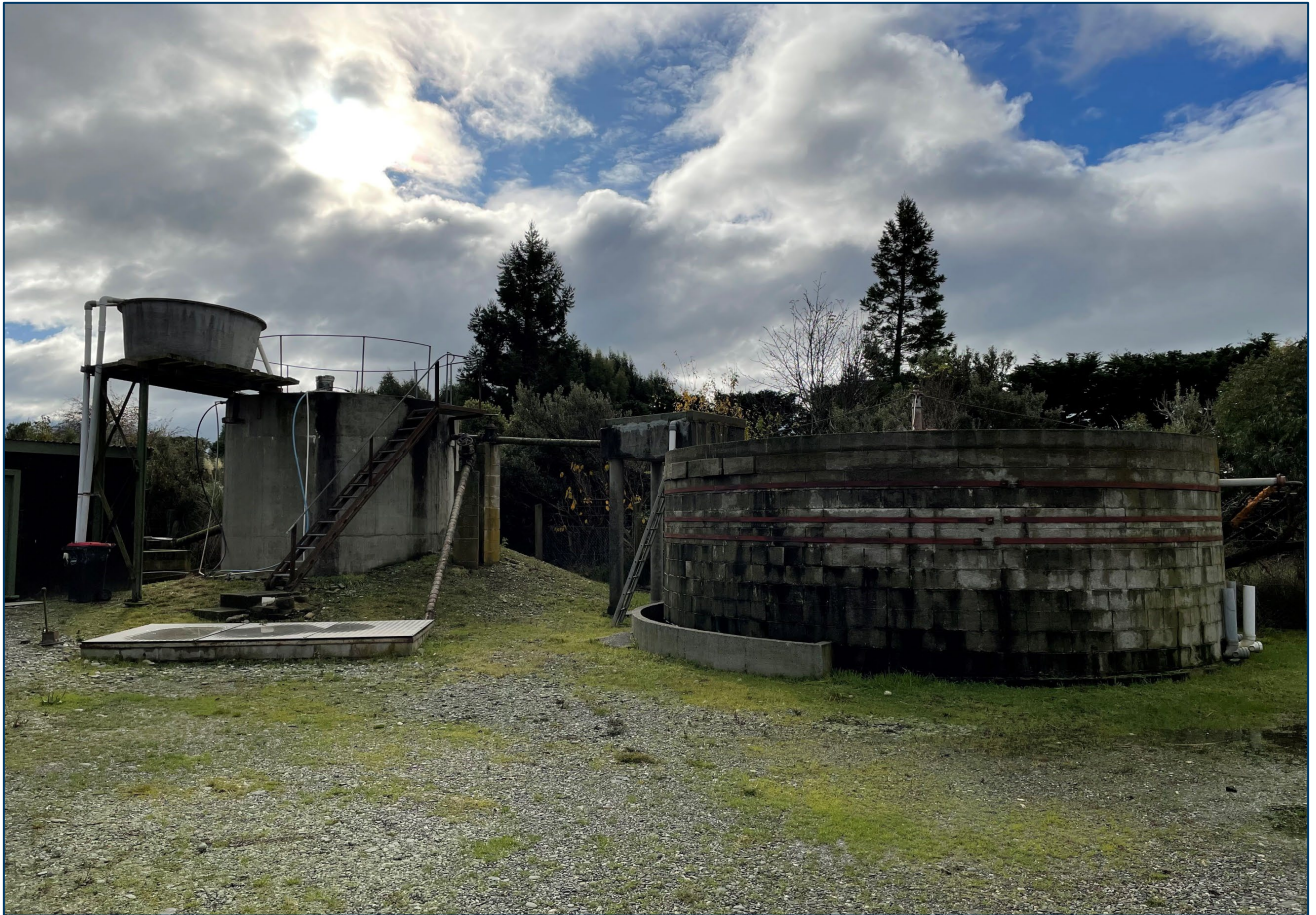
Figure 2 Balfour existing WWTP
