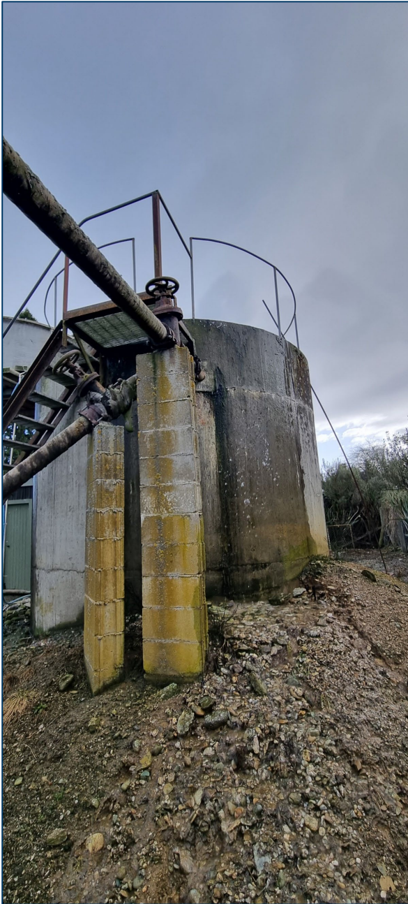
Figure 35 Imhoff tank wet weather overflow
