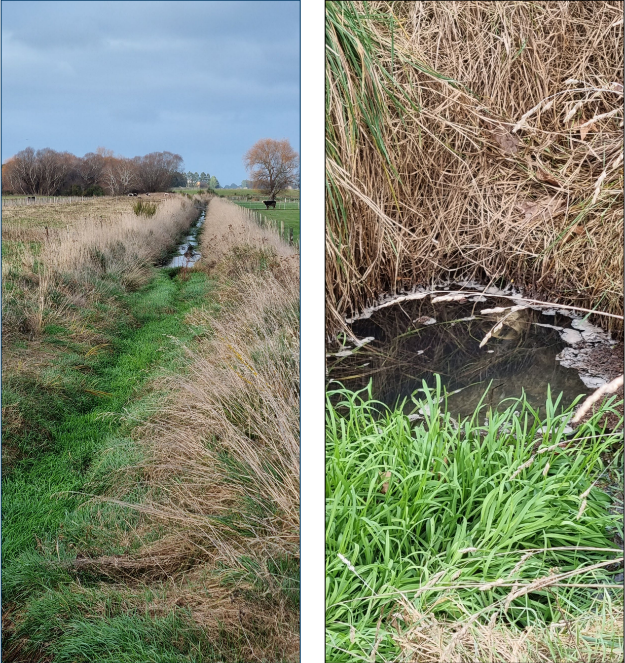
Figure 8 Weeded Drainage Channel and wastewater (left) Wastewater mains outfall pipe into Weeded channel (right)
