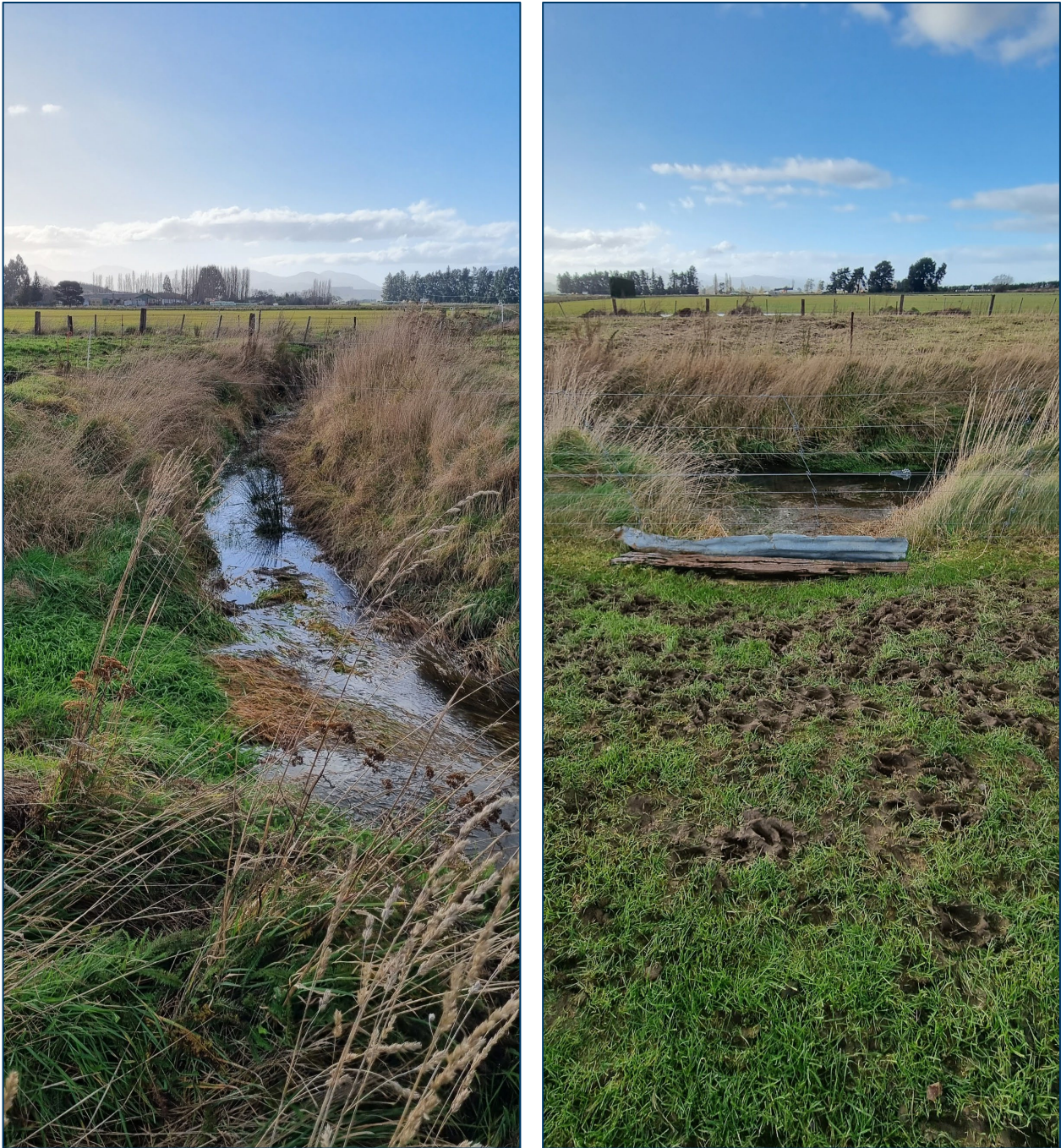
Figure 9 Stormwater inflow through farm drainage channel (left) Overland inflow from neighbouring property (right)
