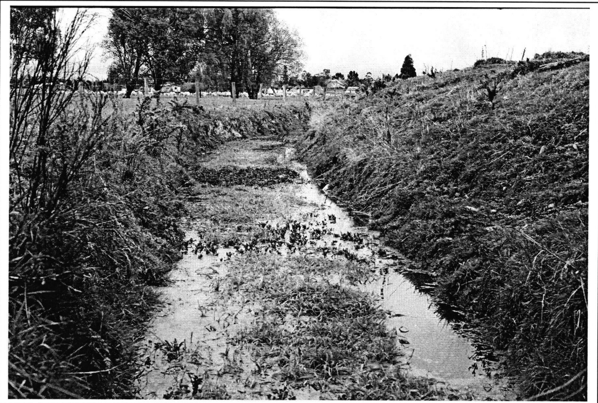
Weeded ditch near discharge point to Longridge Stream
