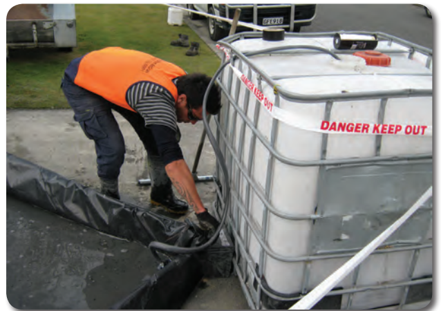
Pumping washwater into a tank for safe disposal (Photo: Environment Canterbury)
