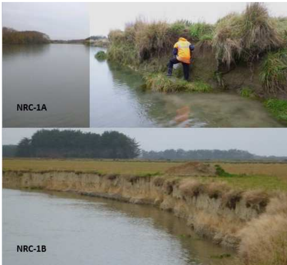
Figure 9: Extensive bank erosion on the Oreti River. NRC-1A shows the erosion on the true left bank upstream of Wallacetown; NRC-1B shows erosion on the true right bank between Wallacetown and the Makarewa River inflow. [Photo date 22/05/2013].
