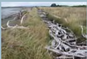
Driftwood filled drain parallel to the eastern shoreline.
