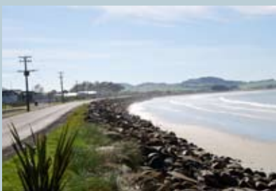
Rock seawall Colac Bay
