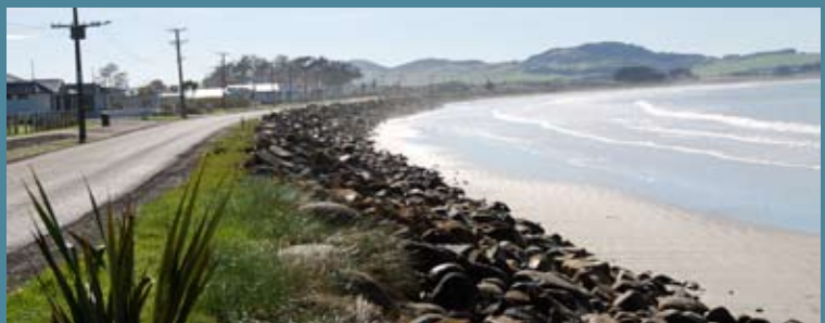
Colac Bay seawall.
