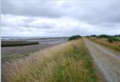
Seawall in Waihopai Arm, New River Estuary
