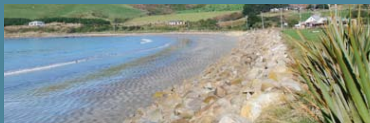
Colac Bay seawall.
