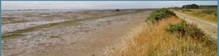
Seawall and stopbank, road on one side and muddy estuary on other - reclaimed section of New River Estuary.
