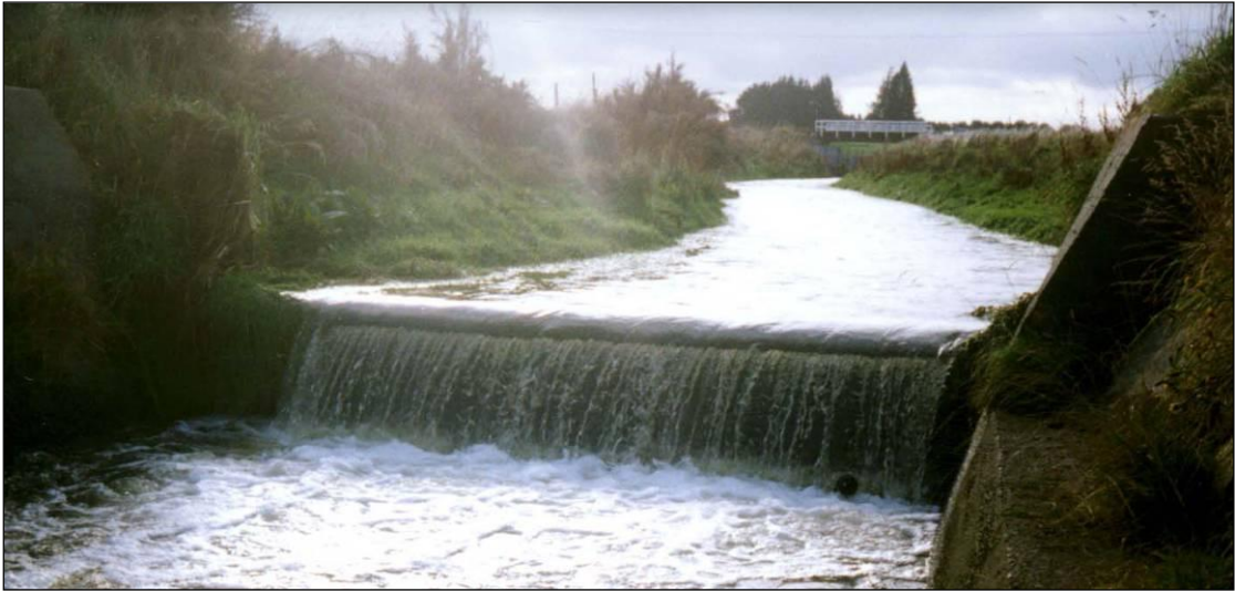
Figure 13: Photograph of one of the Oteramika Creek drop structures (source: Hamill, 1998)
