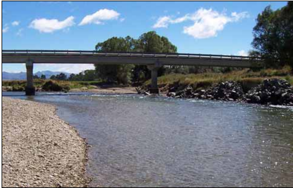
Figure 29: Looking upstream the Waikaia River at the Waipounamu bridge
