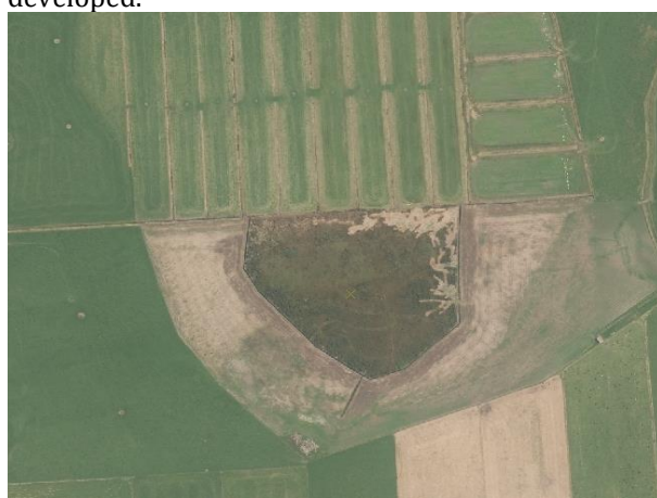
C. 2014 aerial photo. Exotic shrubland cleared, new drain will progressively dry out remaining bog and gorse will reinvade allowing eventual clearance without requiring consent.
